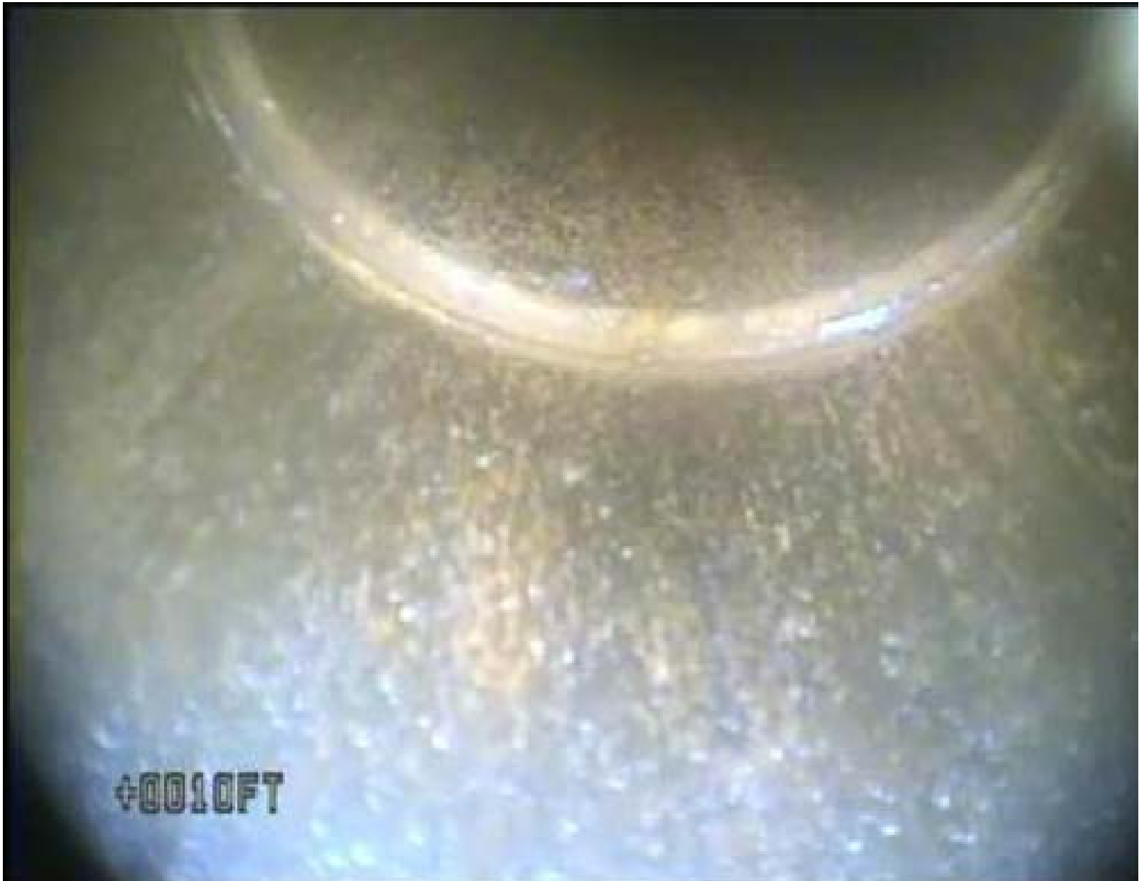
Casing joint not completely connected.
