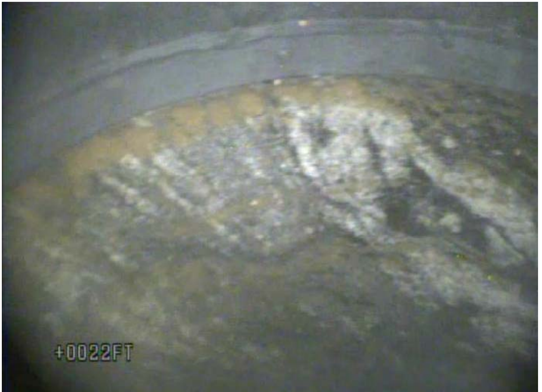
Casing on Bedrock – Below Water
