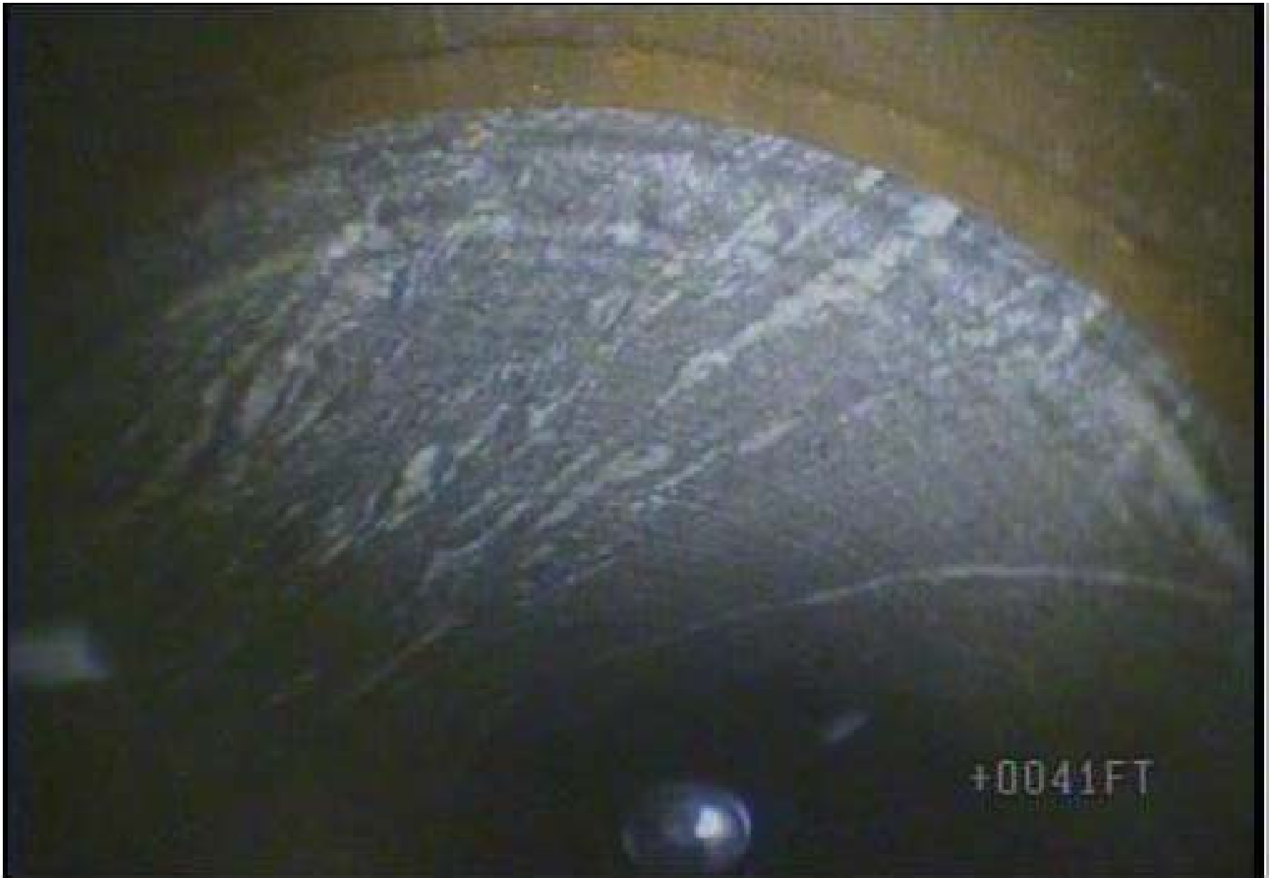
Casing on Bedrock - Above Water
