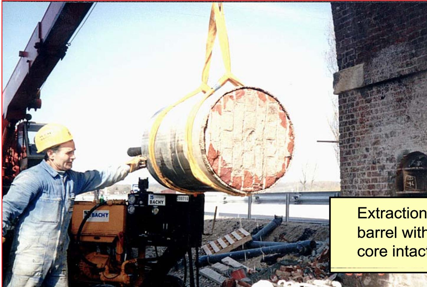
Extraction of core barrel with brickwork core intact
