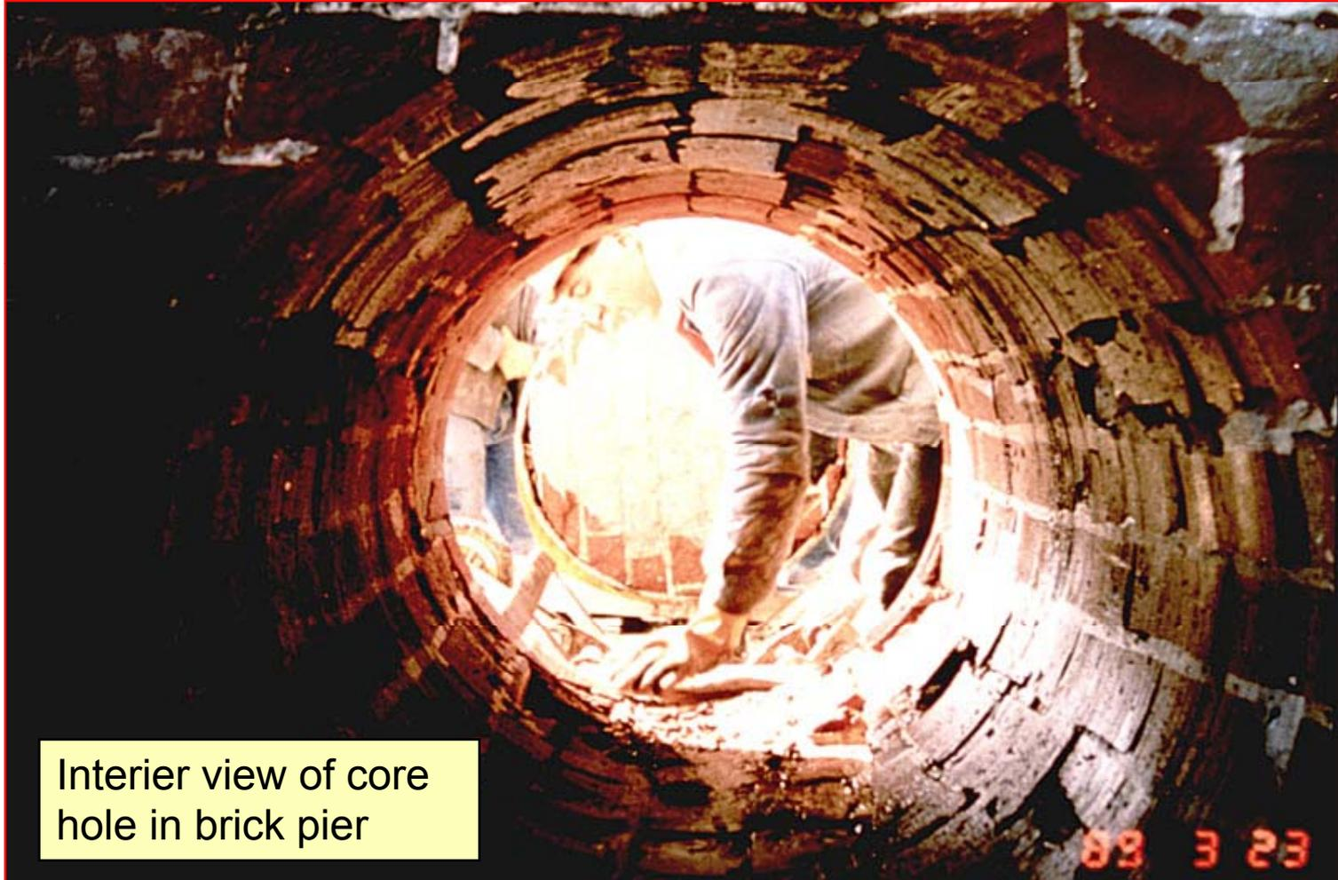
Interior view of core hole in brick pier
