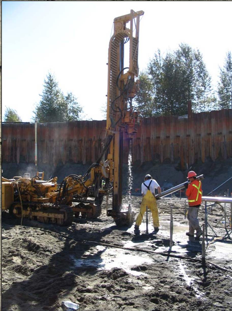
Drill string advancement
