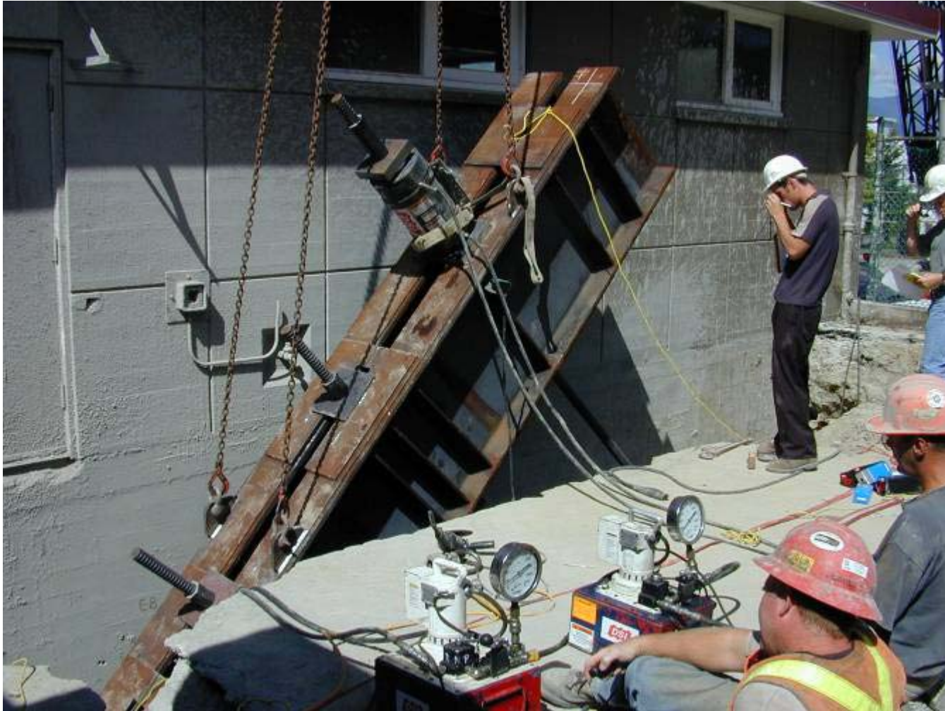
Inclined Compression load testing of production GEWI-Piles
