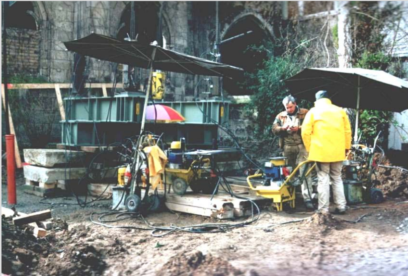
pile test equipment
