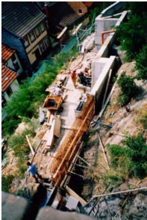
Wall panels from above
