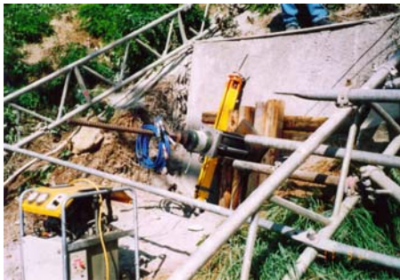
Static load test
