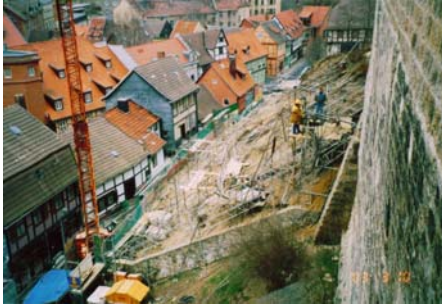
Anchor drilling
