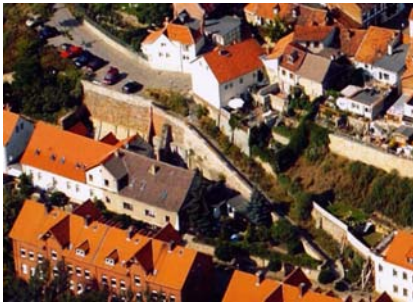
General view after finish
