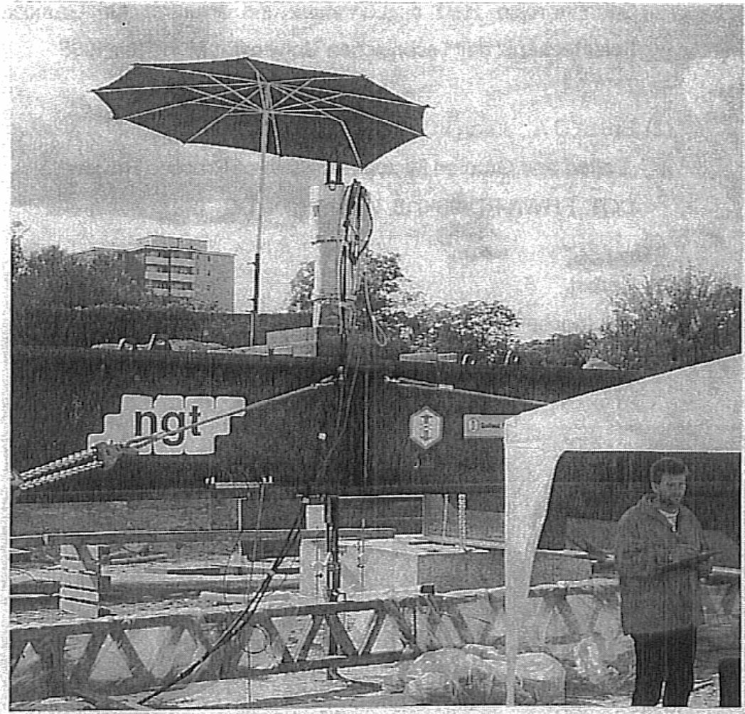
Fig. 8 Pile group test near excavation
