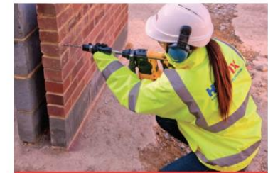
DryFix tie being power-driven into pilot hole
