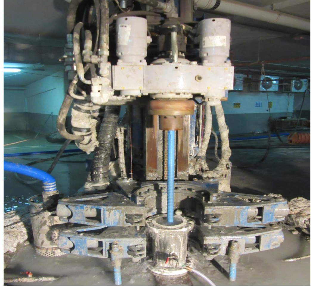
Figure 7: Start to install the hollow bar
