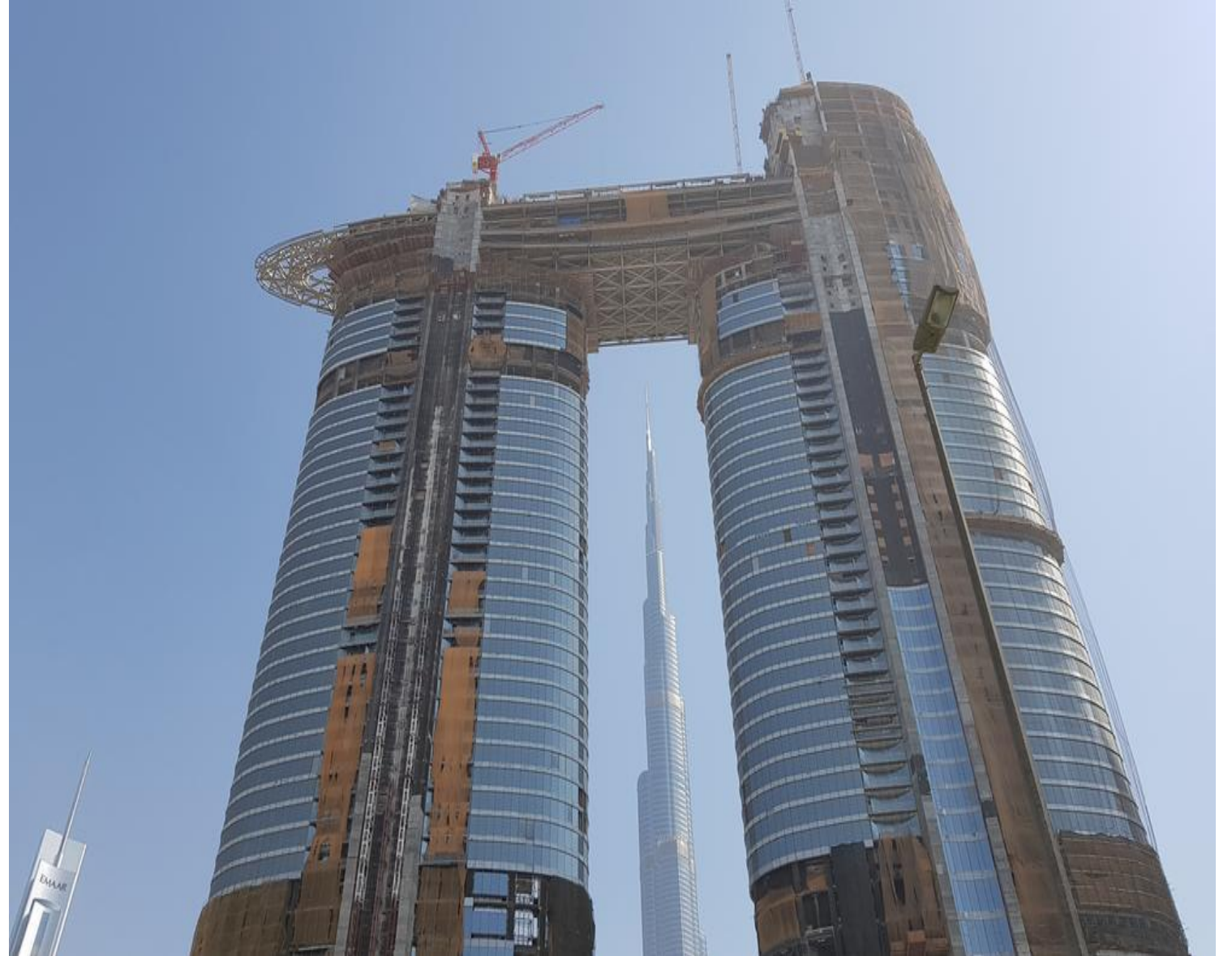
Figure 29: Sky View Tower under construction
