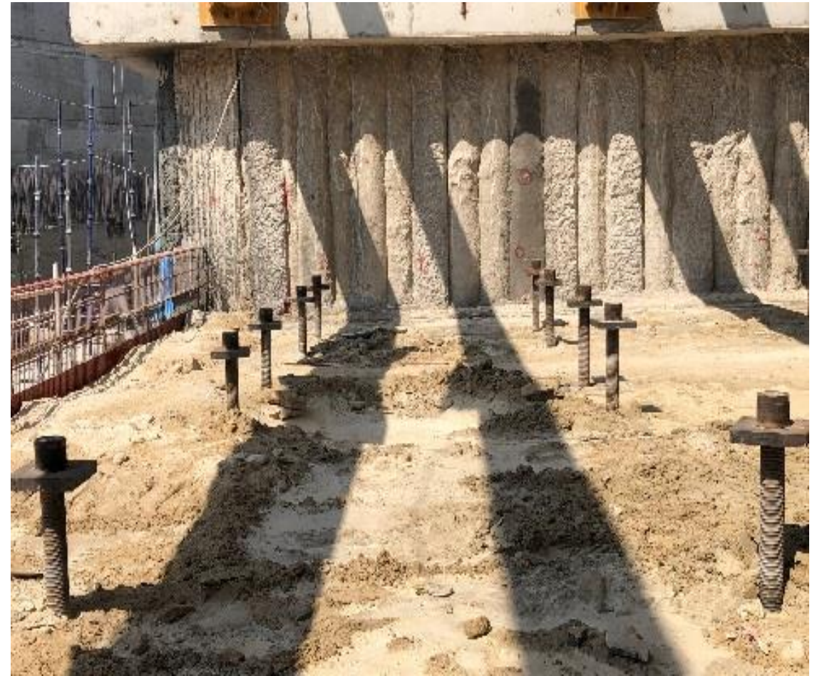
Figure 26: Piles completed
