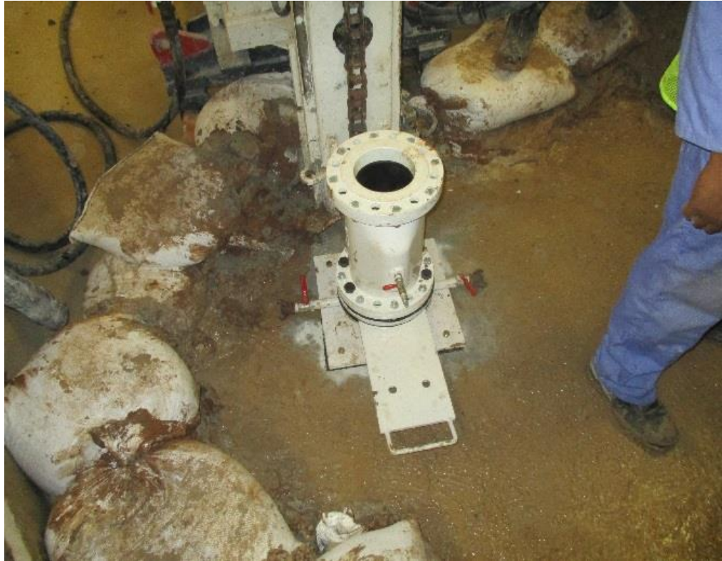
Figure 17: Preventer installed
