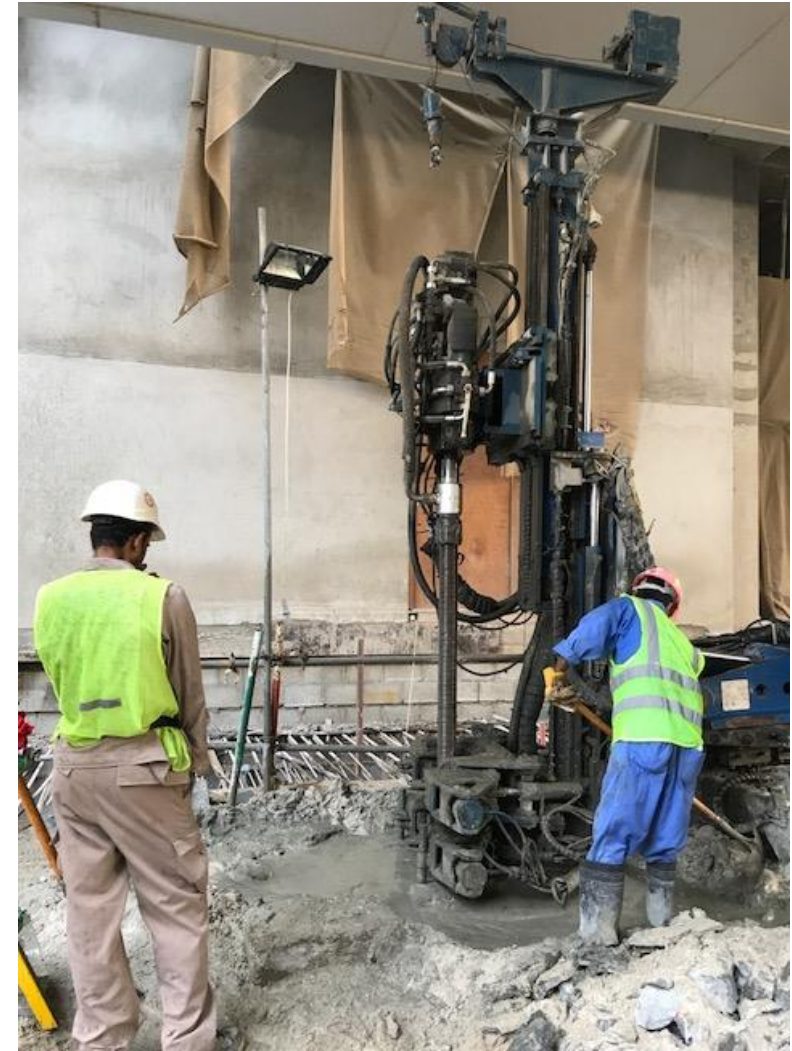
Figure 31: drill rig underneath the metro traveller
