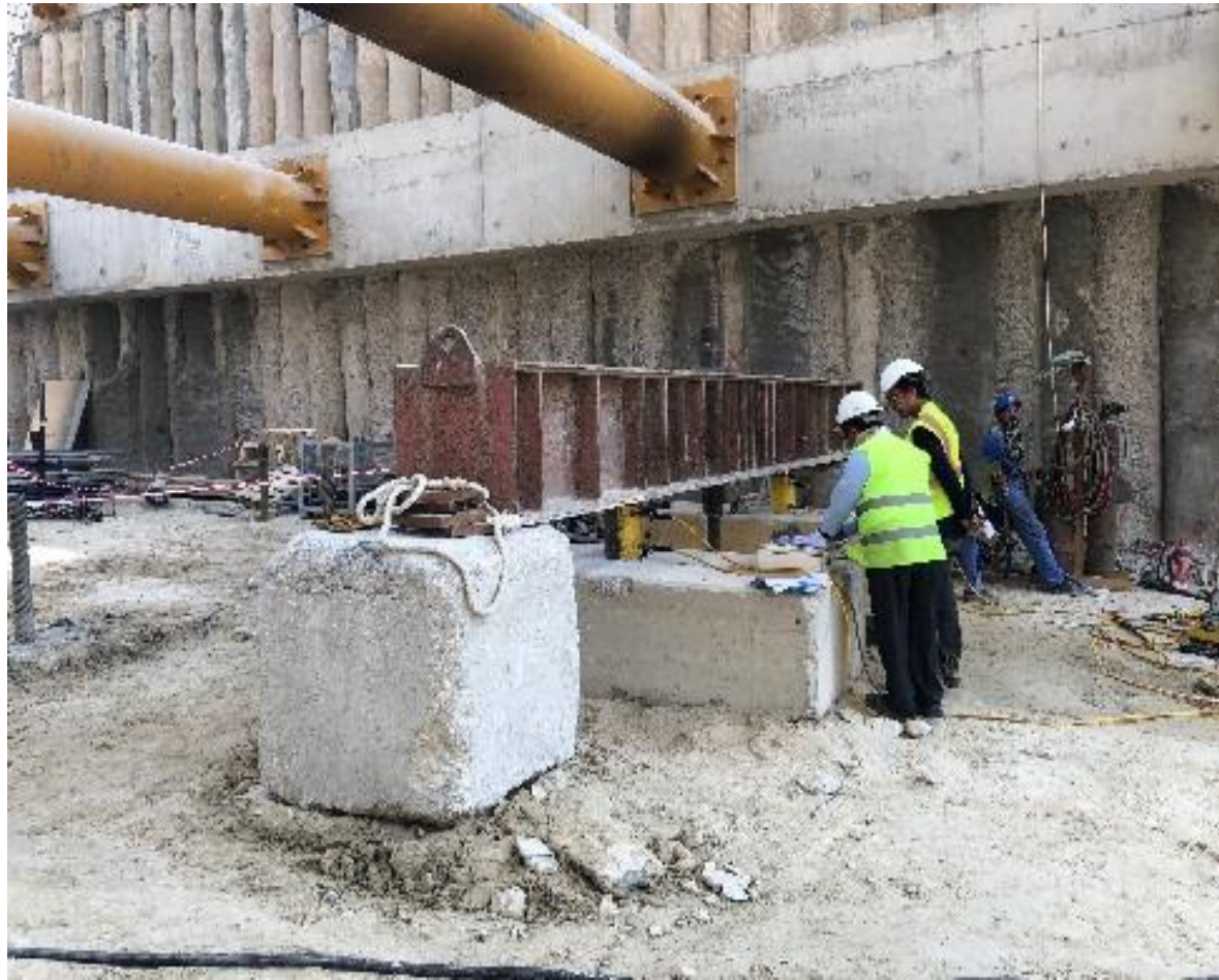
Figure 25: Pile testing set up
