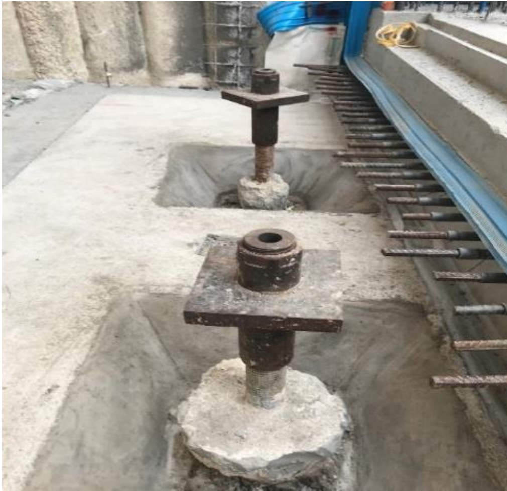
Figure 27: blinding, pile heads, connecting dowels, water stopper
