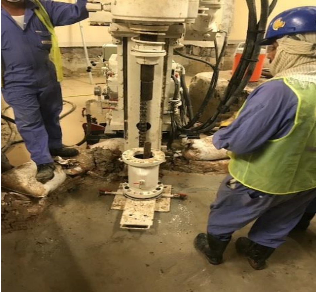
Figure 18: First Bar almost fully installed
