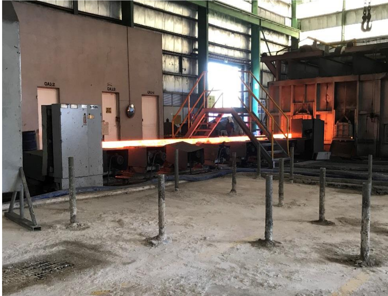
Figure 38: piles on the ground floor after execution
