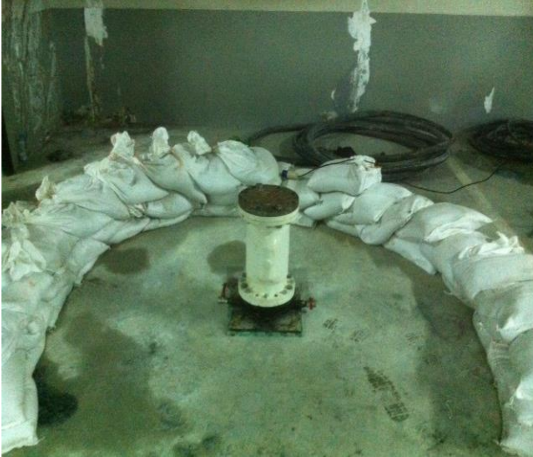
Figure 6: Preventer is installed
