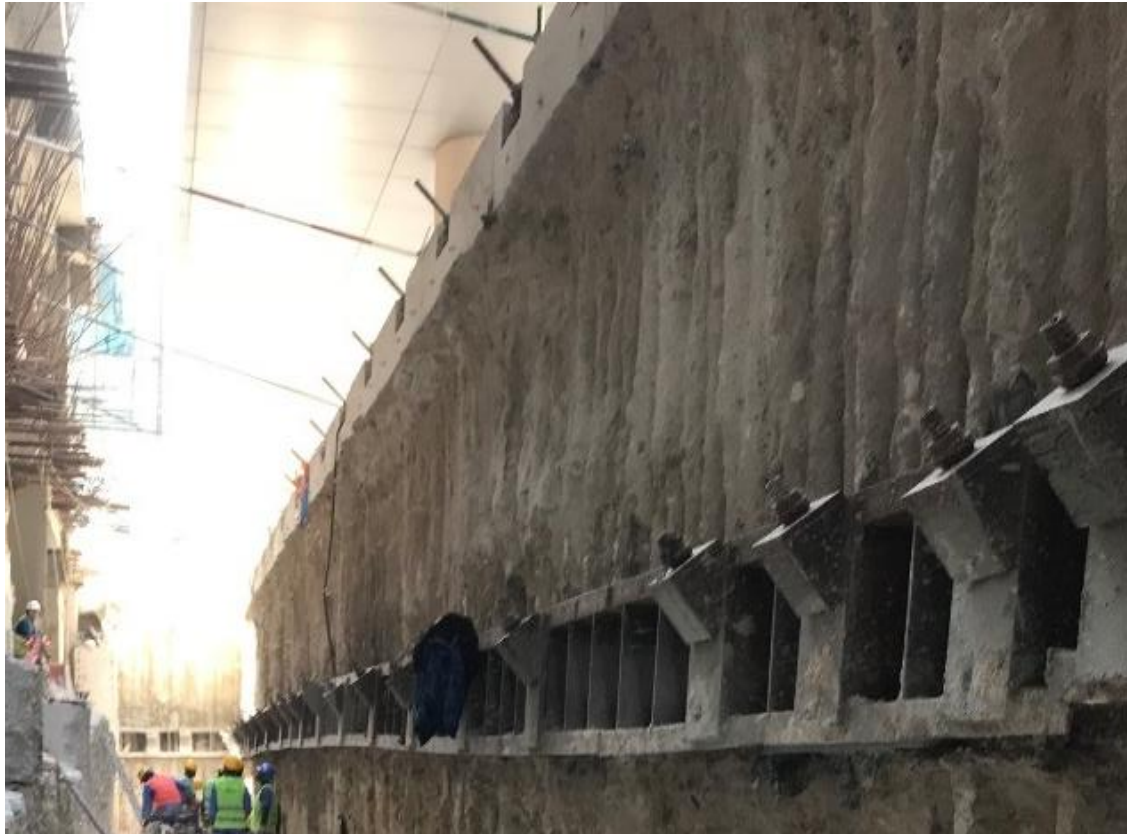
Figure 32: temporary shoring wall
