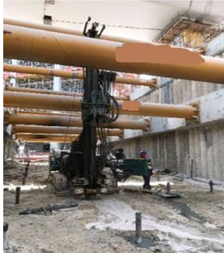
Figure 24: Drilling underneath fully operational road
