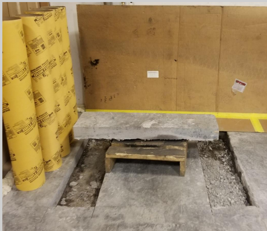
Cut out of concrete pad
