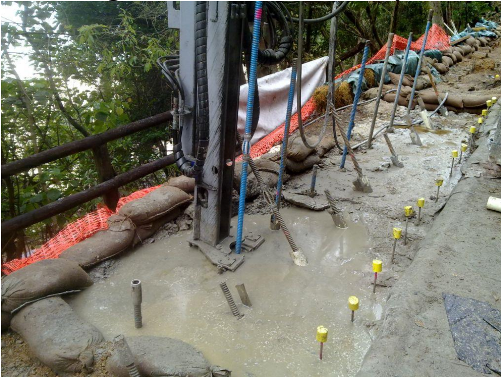
Drilling of TITAN Hollow bar piles
