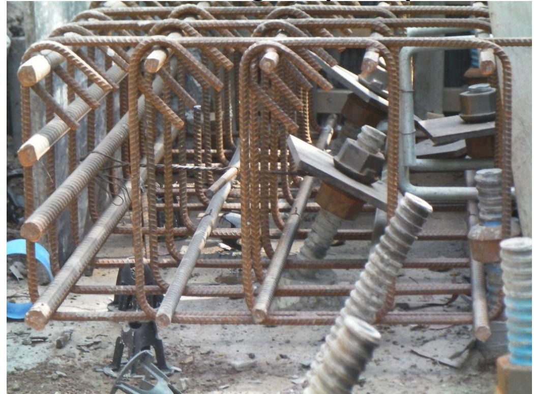
Reinforcement cage of pilecap beam
