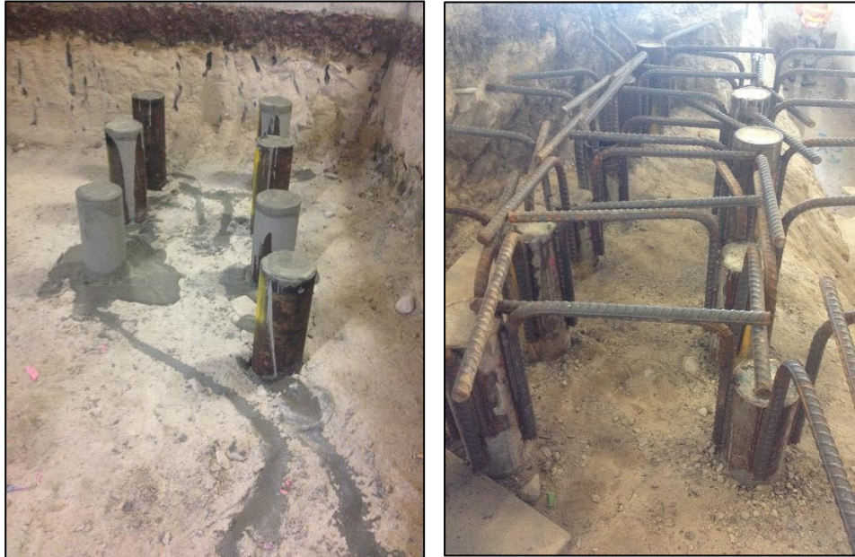
Figure 10. Grouted steel tube micropiles in NE core
