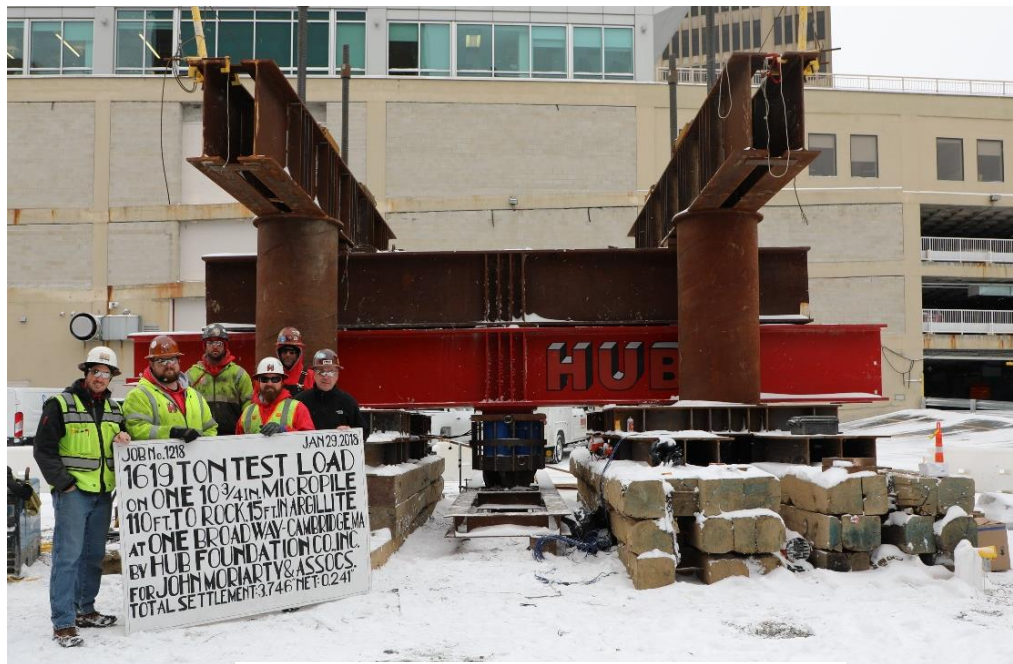
Photo 10: 1619 Ton Pile Load Test on Micropile Performed on Site
