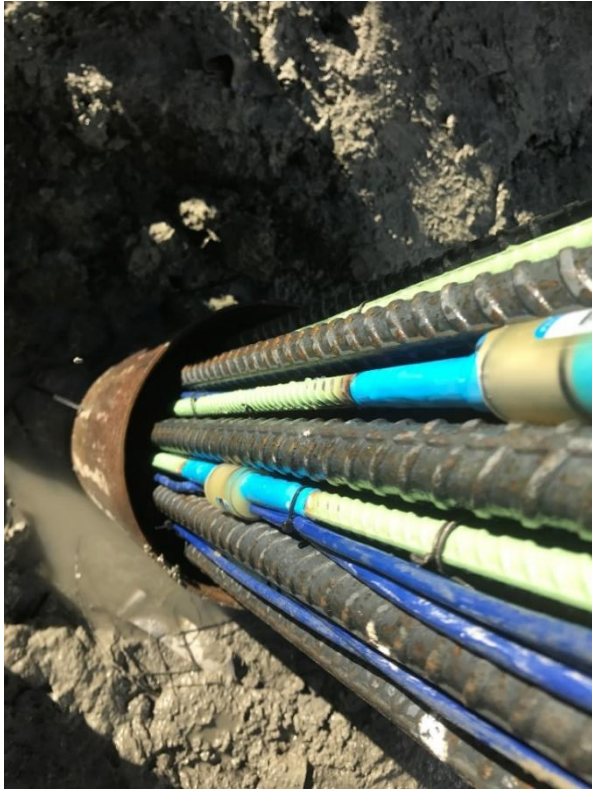
Photo 1: Test Pile Socket Reinforcing and Instrumentation
