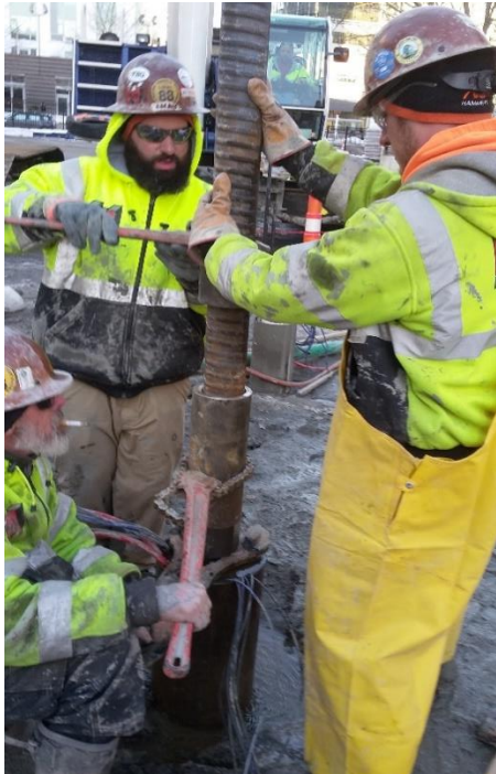
Photo 3: Threading together No.32 Bars
