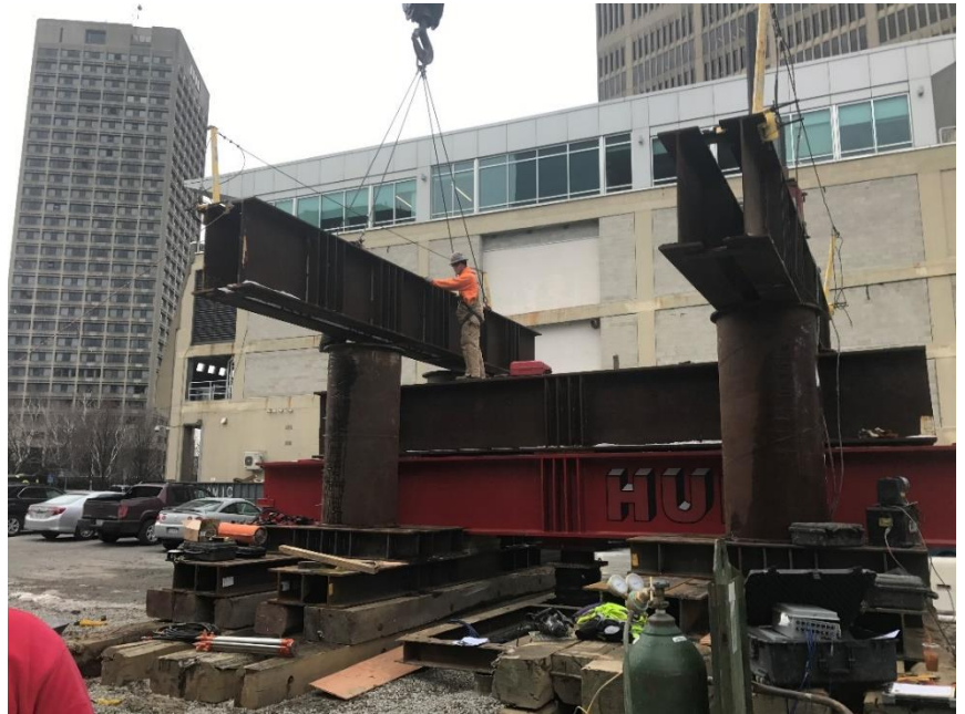
Photo 4: Constructing the Test Frame
