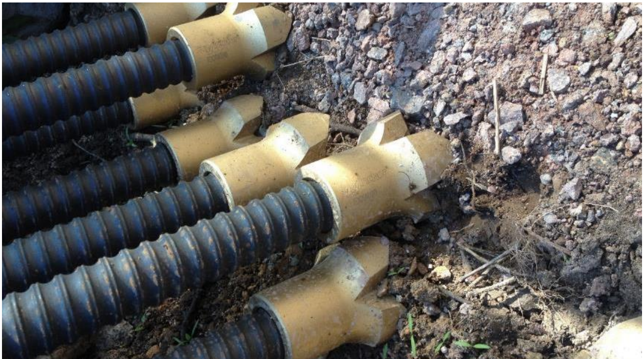
Photograph 1. Sacrificial cutting shoe attached to the toe of each micropile
