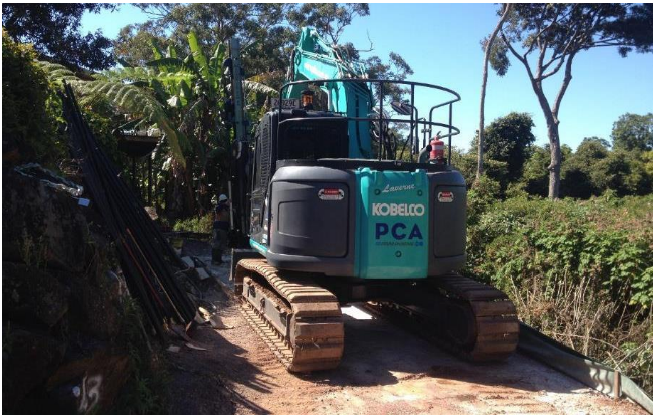
Photograph 3. Micro-piling commencing at eastern end of Bay 3
