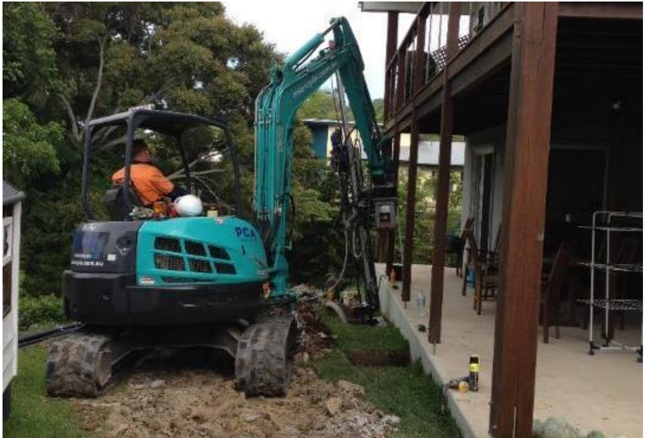
Photograph 8. Underpinning in progress on southern side of house
