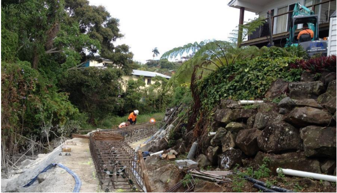
Photograph 9. Capping beam reinforcement being constructed
