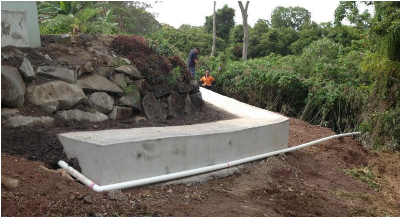
Photograph 10. Completed capping beam. View south-east
