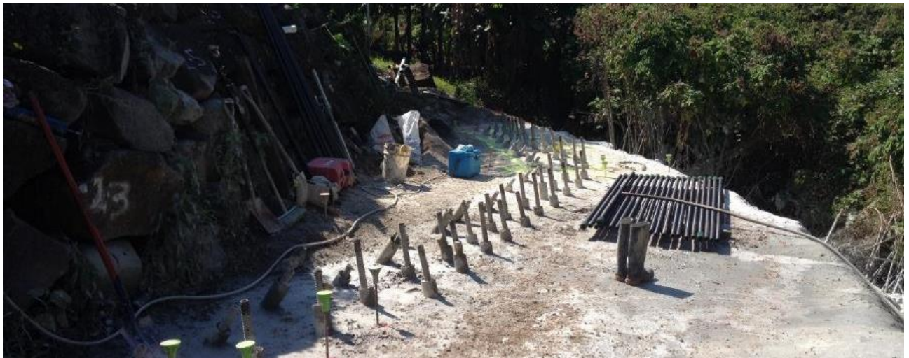
Photograph 6. Micropile progress in Bays 2 and 3
