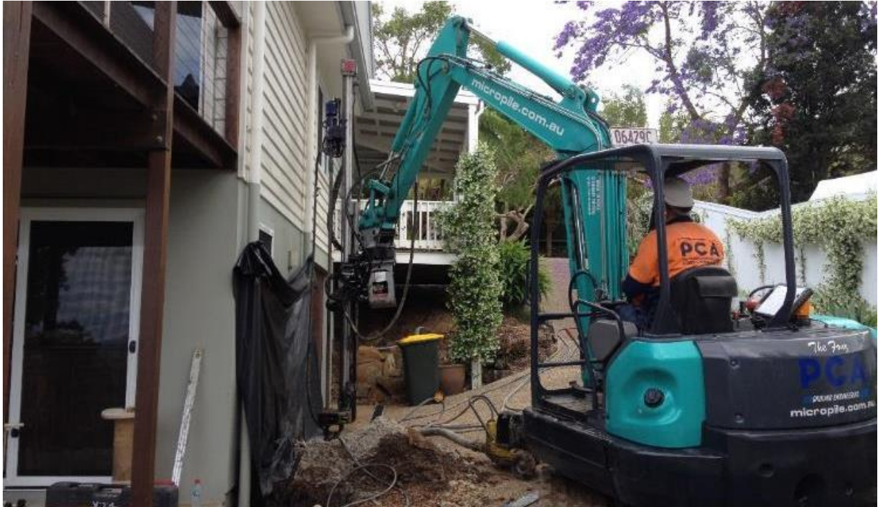
Photograph 7. Underpinning in progress on eastern side of house
