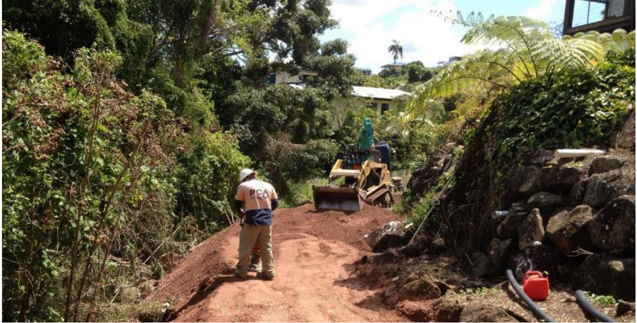
Photograph 2. Construction of piling platform below boulder wall
