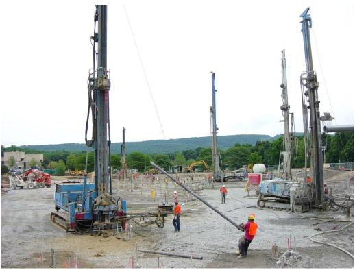
Figure 4. Photo – Large long-mast rigs make greenfield applications cost effective.
