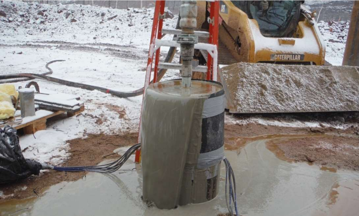
Figure 10: Completion of grout placement.
