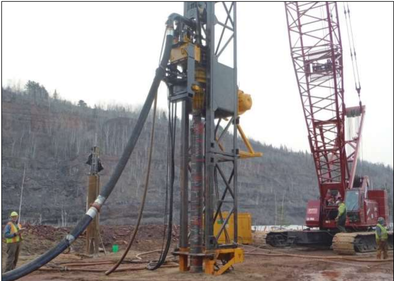
Figure 6: Test pile installation.
