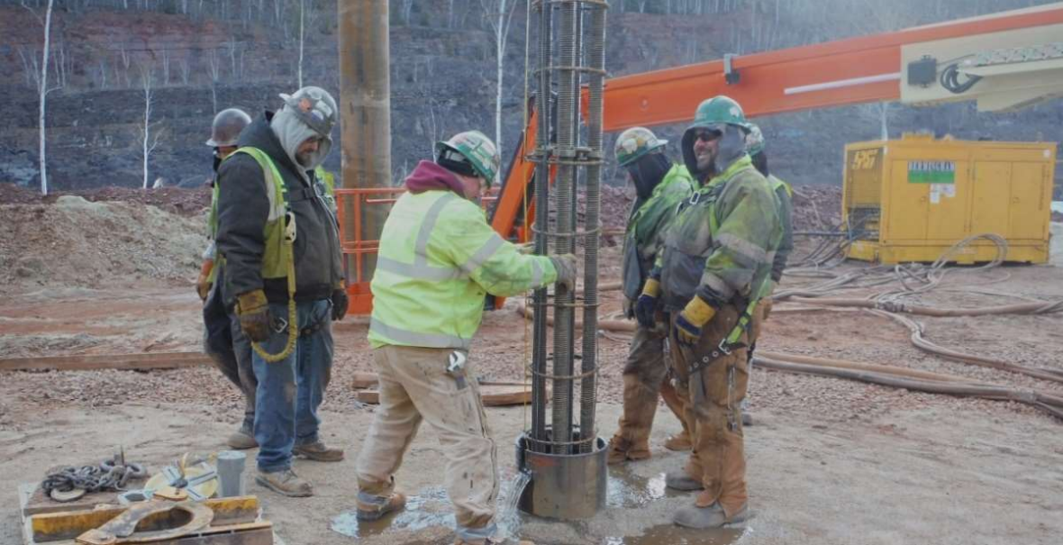
Figure 9: Installation of reinforcing cage.
