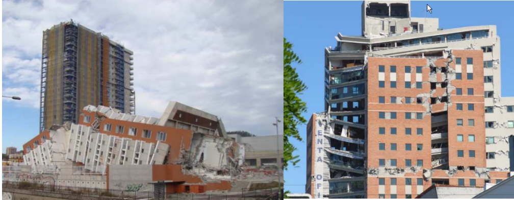
Figure 5 – Alto Rio Tower (fully collapsed, left) and O'Higgins Tower (partially collapsed, right) [2]
