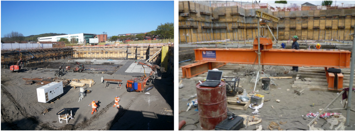
Figure 11 – Installation of the micropiles (left) and load tests (right)
