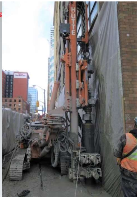
Figure 9. Drilling against the Façade
