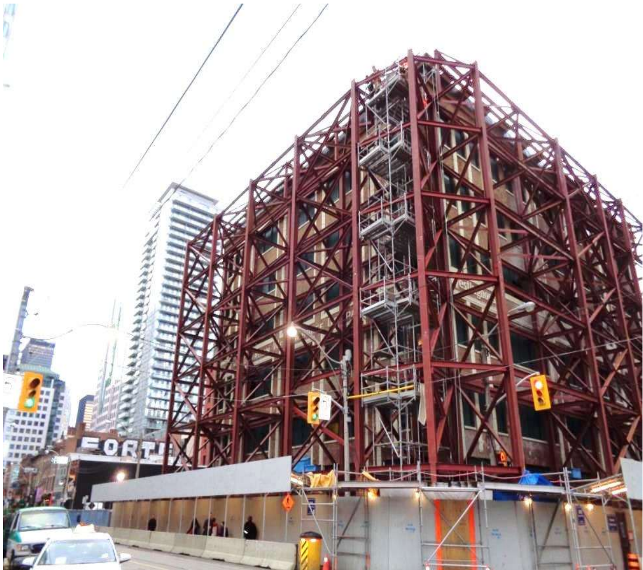
Figure 4. Façade Support Frame
