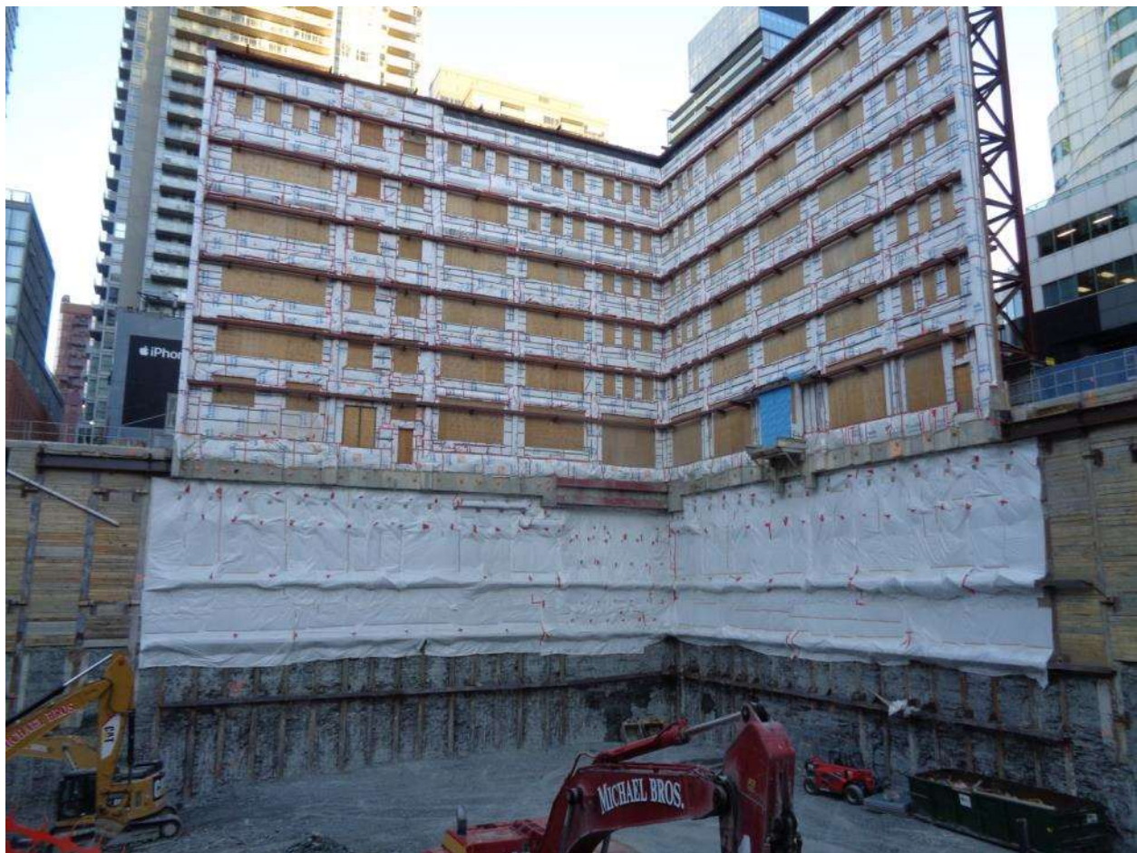
Figure 13. Frost Protection under the Façade
