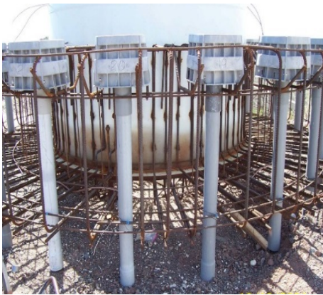
Figure 15. Pre-set sleeves in footing
