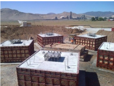
Figure 11. Ready for post-tensioning
