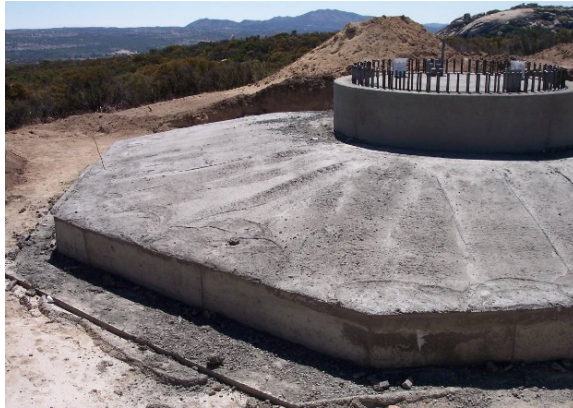
Figure 2. Large reinforced concrete spread footing, with 500 to 600 cy of concrete
