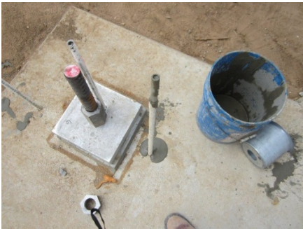
Figure 14. Finished grouting the GVF
