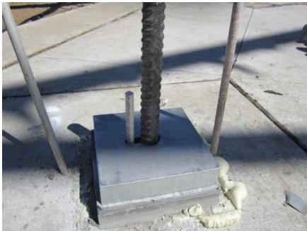
Figure 12. Bearing plate with grout tubes
