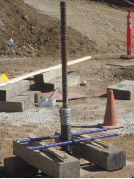
Figure 8. Placing bar and grouting
