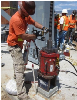
Figure 13. Stressing of solid bar tendon
