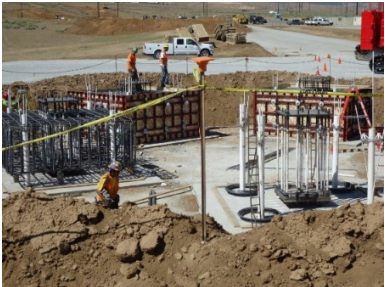
Figure 10. Placing rebar and forms
