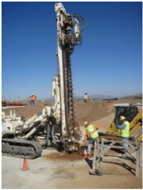
Figure 7. Drilling lager hole
