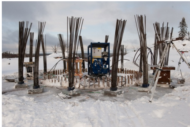
Figure 23. Typical post-tensioned wind turbine foundation with strands
