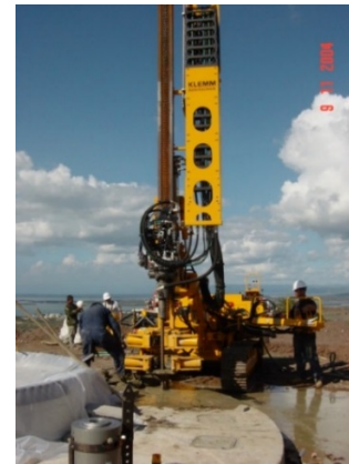
Figure 16. Drilling of a hollow bar
