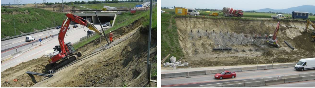
Figure 11 a+b – Slope stabilization on S1 highway Austria
