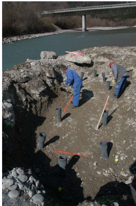
Figure 8 – driven piles – straight and battered
