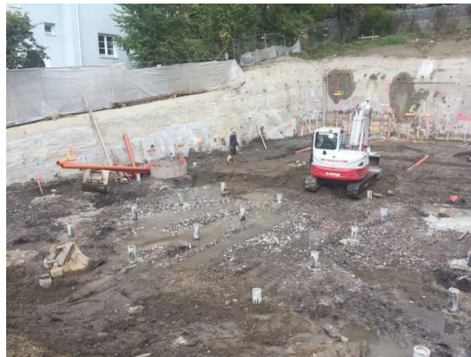
Figure 13 – preparation of foundation level
