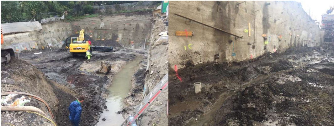
Figure 12 a+b – piling works residential building
