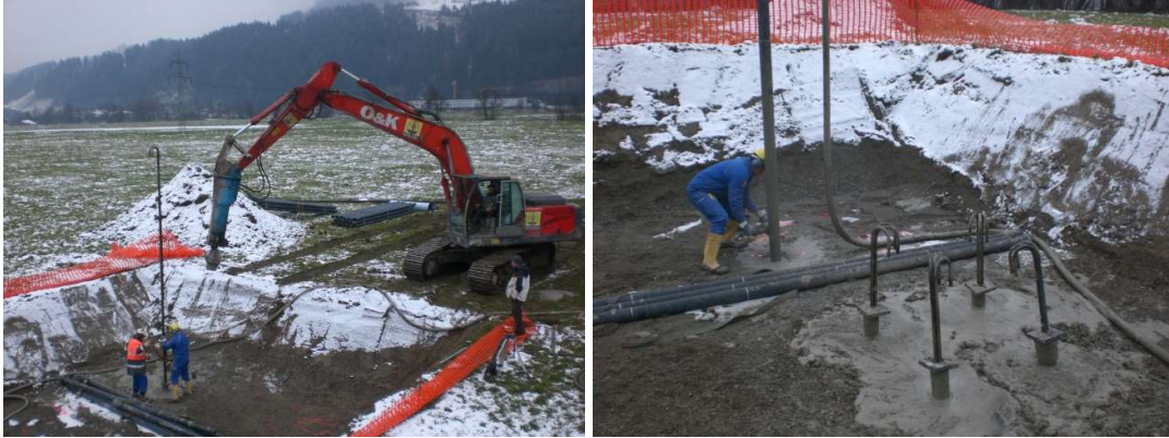
Figure 14 a+b – piling works electric power line HT
