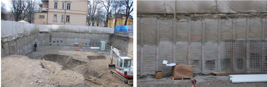
Figure 16 a+b – pit lining piles and shot concrete arches
