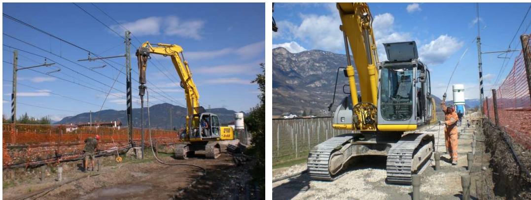
Figure 12 a+b – noise protection wall foundation France
