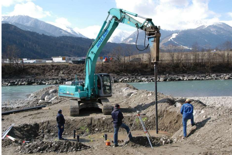
Figure 7 – Pile driving for pier foundation
