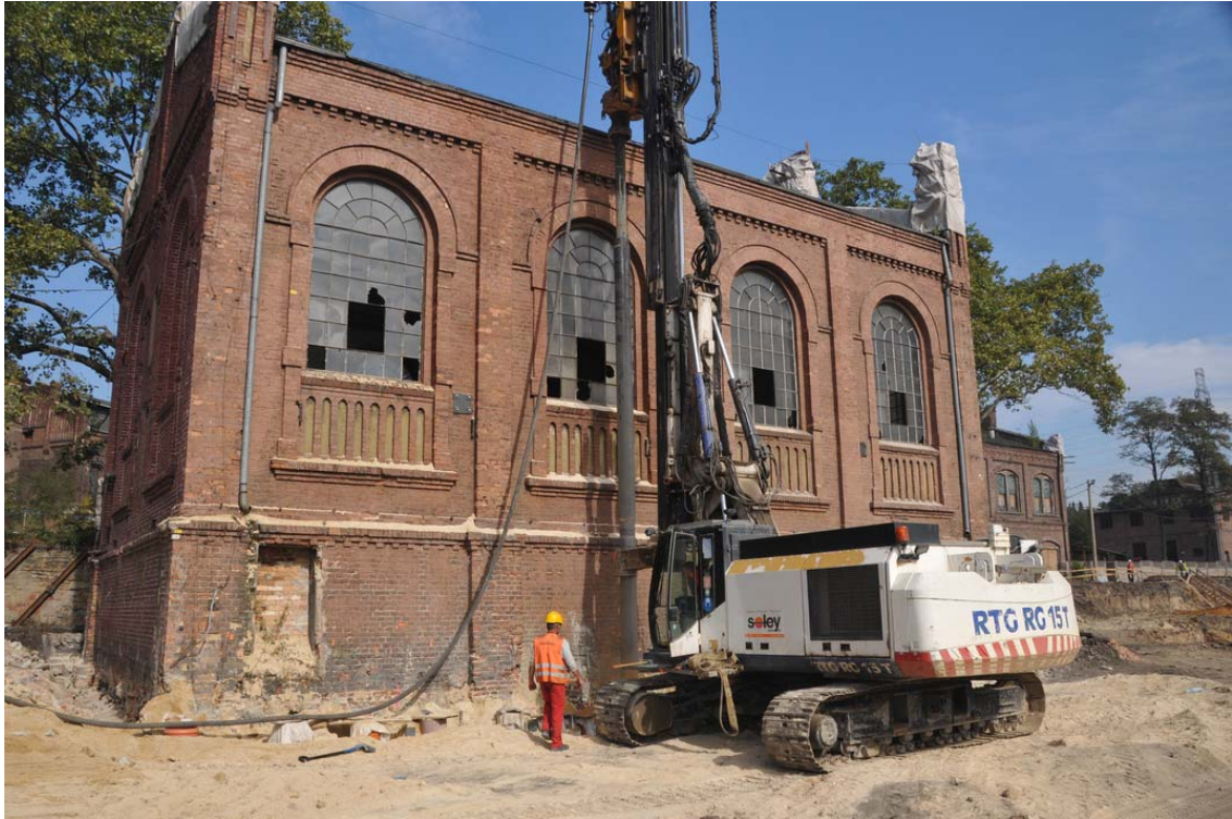
Figure 12. Installation of DFF piles along the walls of building MS-8
