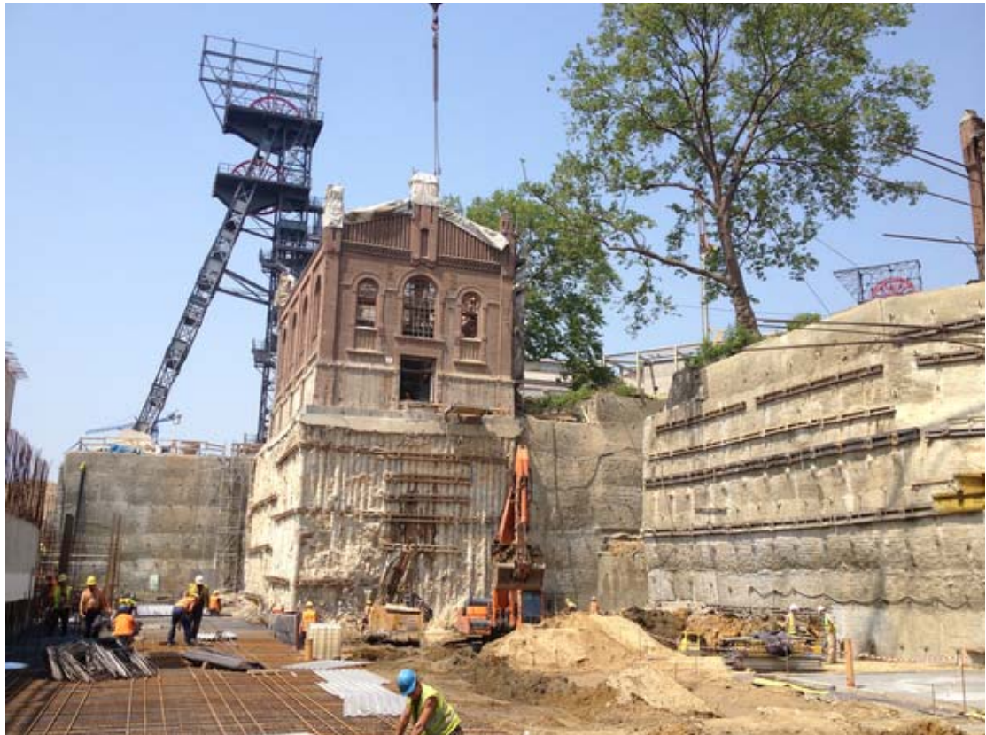
Figure 4. A view towards MS-8 structure and Warszawa shaft
