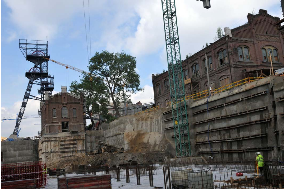
Figure 15. A view of the north wall of the trench with different stabilization
