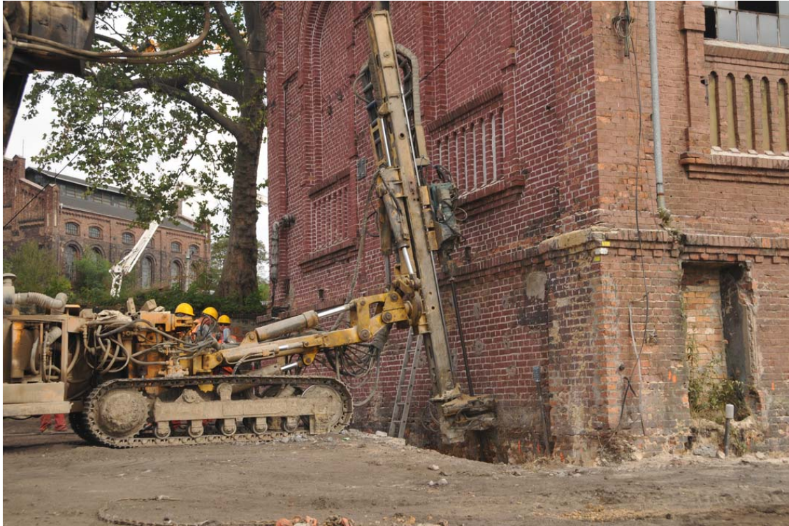
Figure 10. Installation of underpinning micropiles along the building wall
