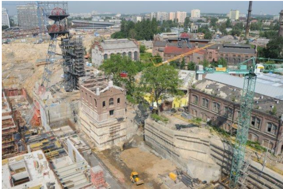
Figure 3. Panorama of the construction site
