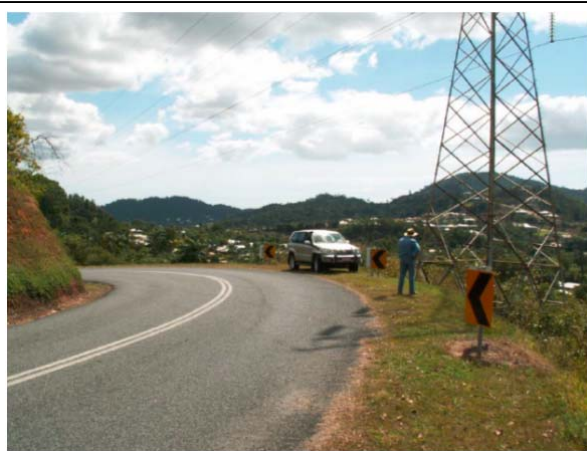
Figure # 3 Tower adjacent to road with sloping access
