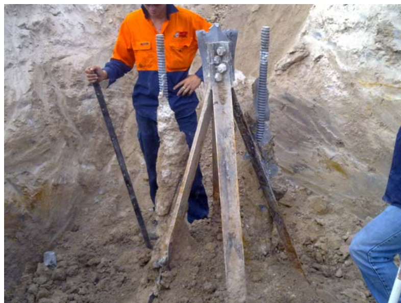
Figure # 9 Micropiles successfully installed within 150mm of the tower leg
