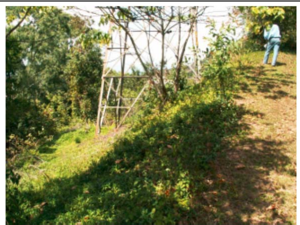
Figure # 4 Tower with steep access in environmentally sensitive location
