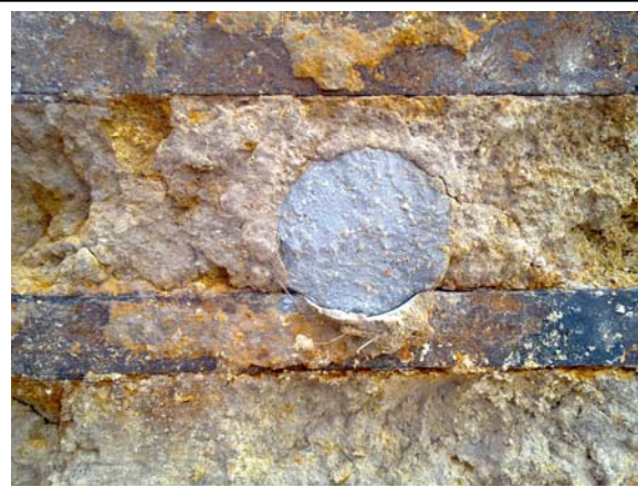
Figure # 8 Exhumed grillage after use of specialist tooling
