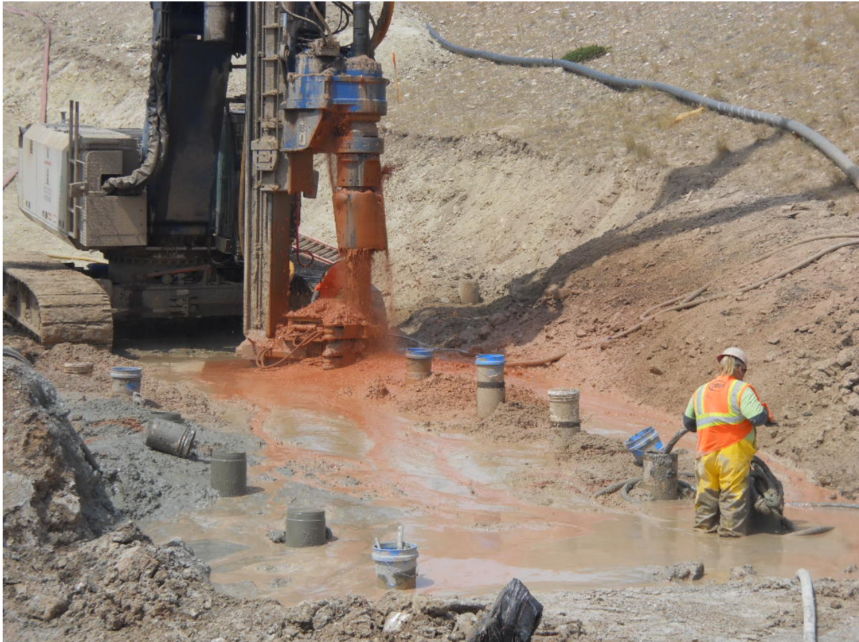
Figure 9. Double Rotary Drill Head
