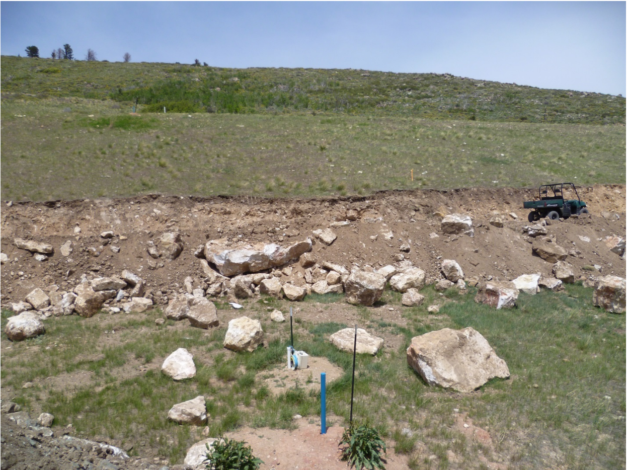
Figure 13. Grading For Drill Benches.
