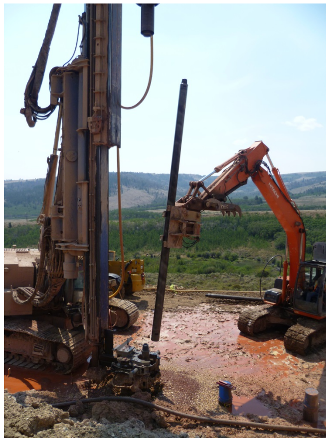
Figure 12. Casing/Drill Rod Handling
