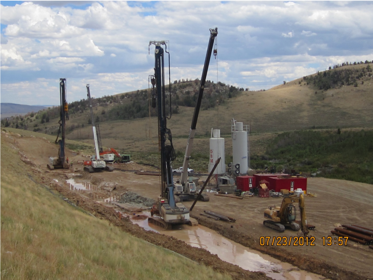
Figure 16. Shear Pile Installation
