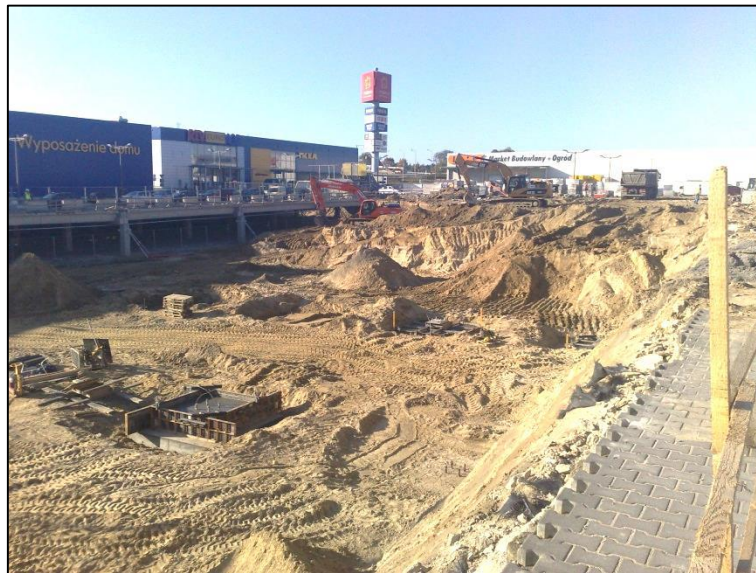
Fig. 10 Earthworks during execution of the underground parking
