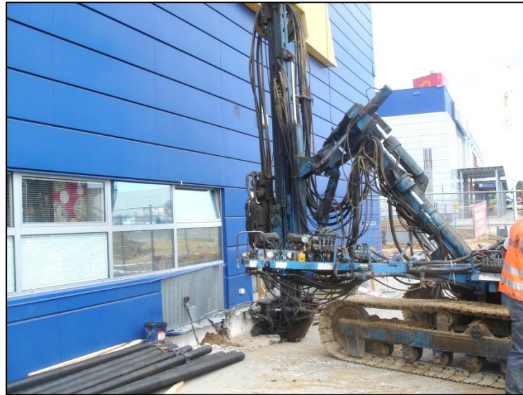
Fig. 8 Executing of the micropiles \Phi=220 mm (Ti103/78 rod),
