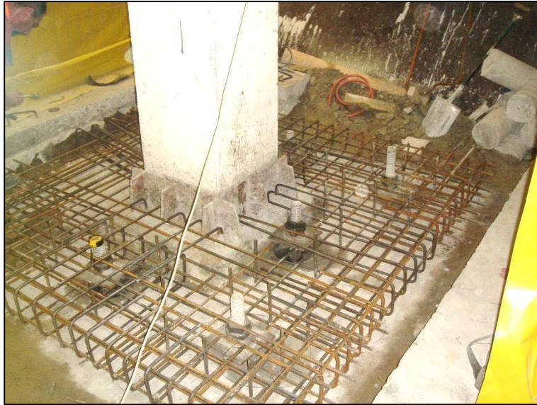
Fig. 4 Micropiles installed in the block of existing foundation
