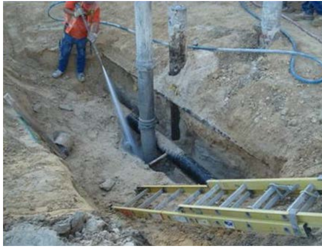
Figure 11. Micropiles surgically installed to clear existing utilities.
