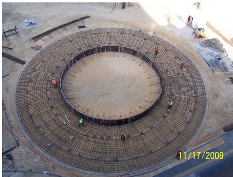
Figure 13. Placement of bottom mat of reinforcing steel and concrete formwork.
