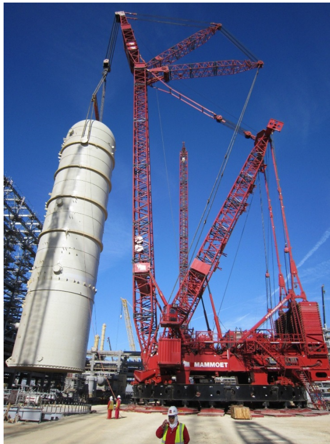
Figure 1. Photo of typical usage and setup for a Mammoet PTC35 ring crane (photo courtesy of Mammoet).
