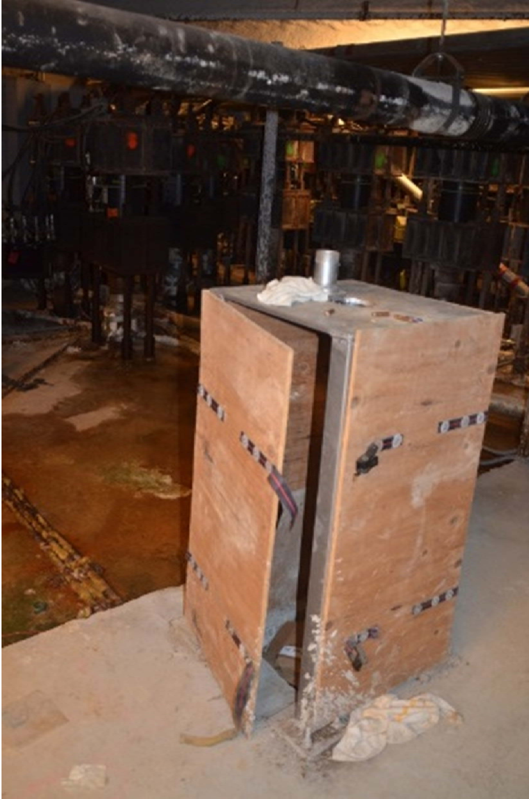
Figure 21 - SONDEX ground deformation monitoring location. Grid point K22 Total depth 210 feet with 94 settlement monitoring depth levels.
