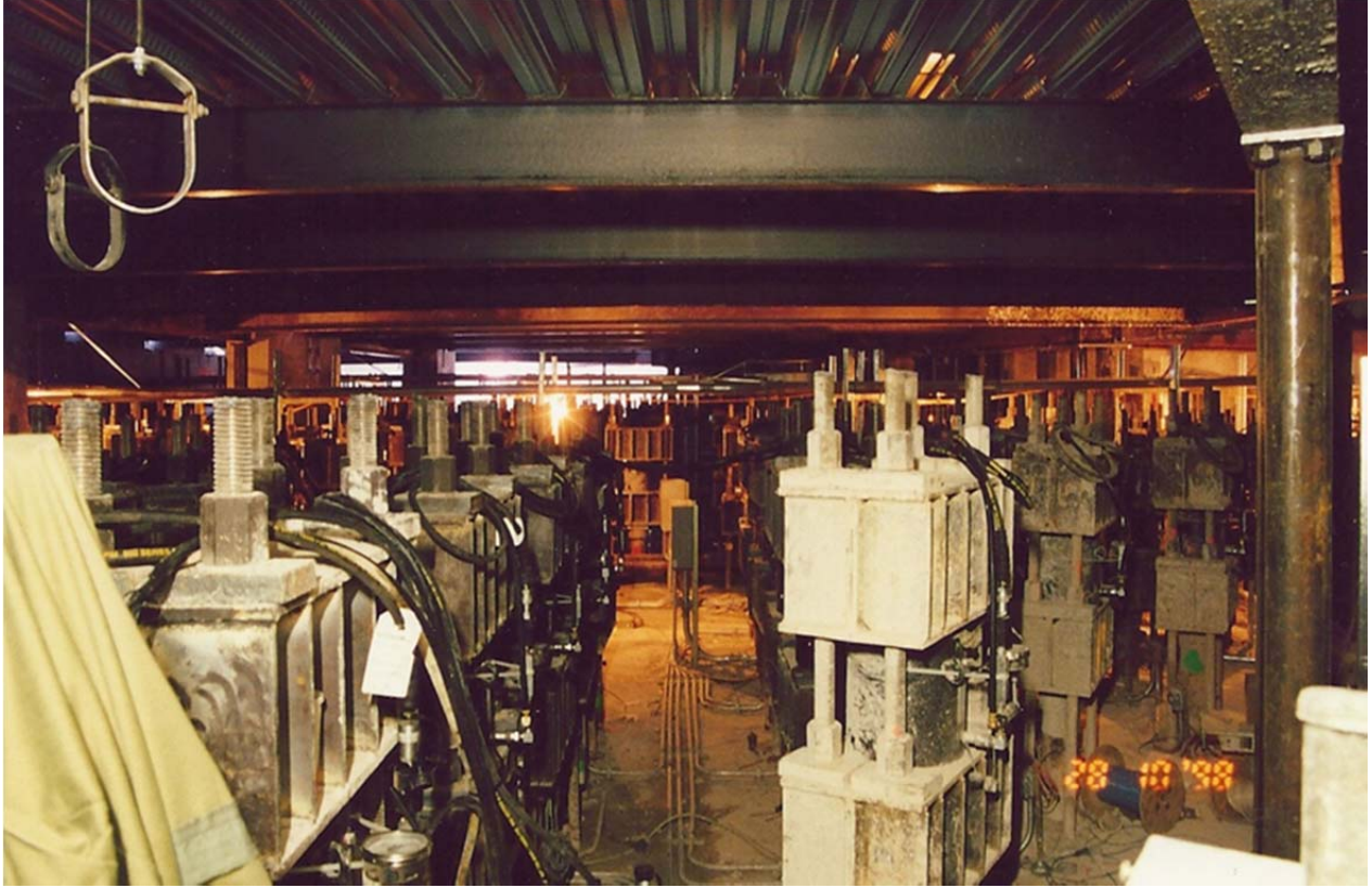
Figure 3 – Between grid lines 27 and 28. Micropile H28 in foreground.
