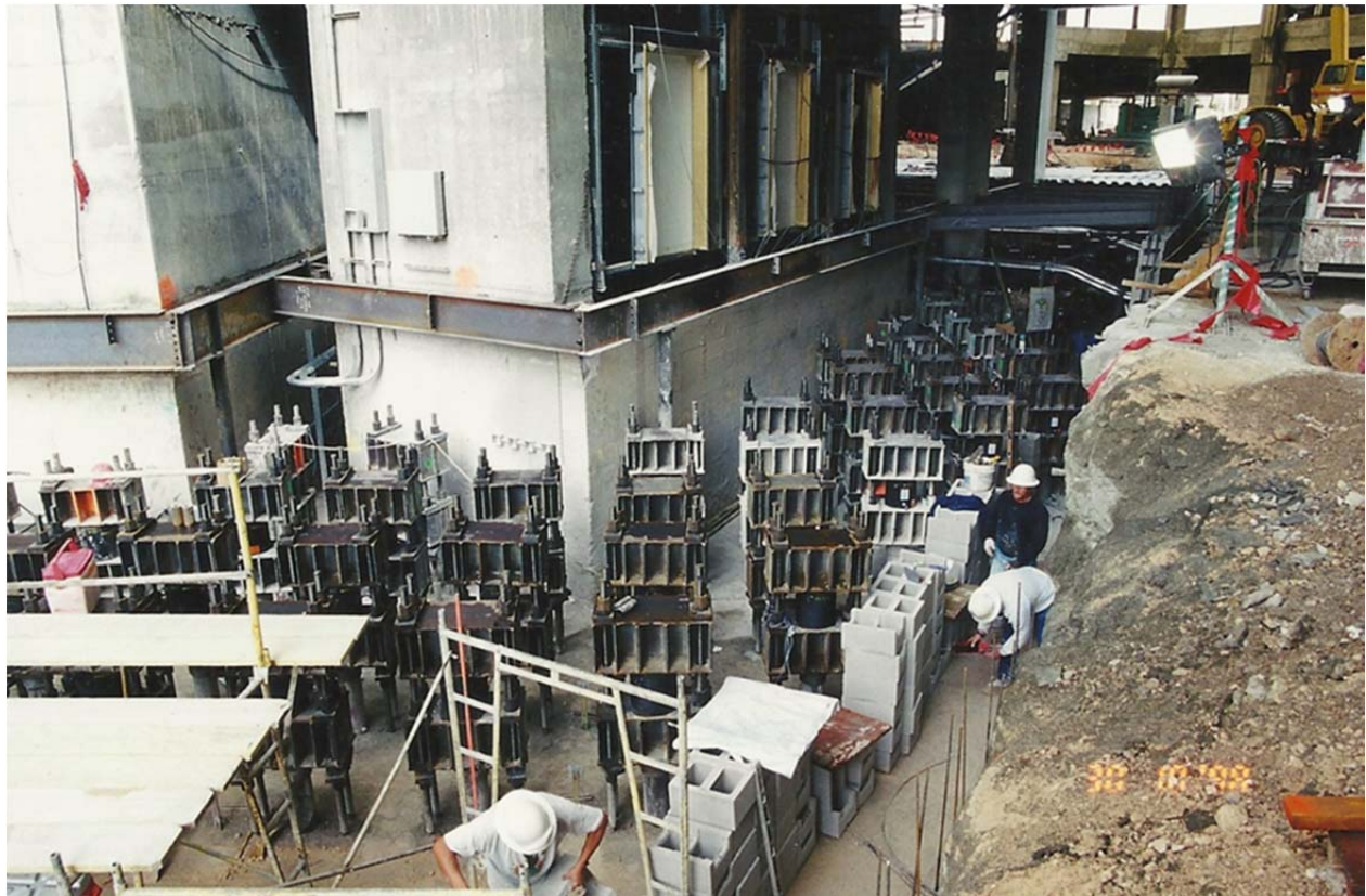
Figure 2 –Micropile installation completed October 9, 1998.
