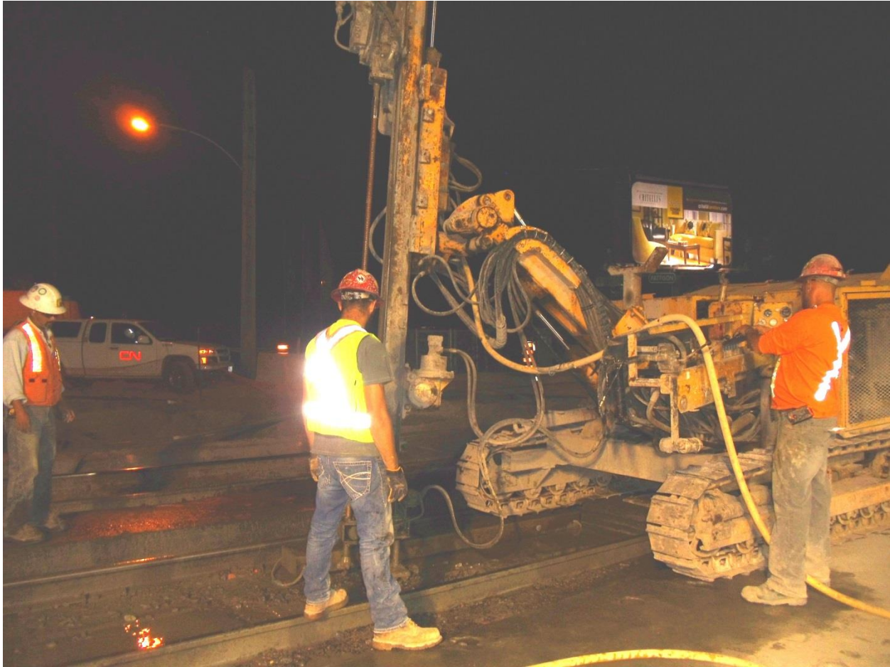
Figure 7: Light weight drill rig installing micropiles during night shift
