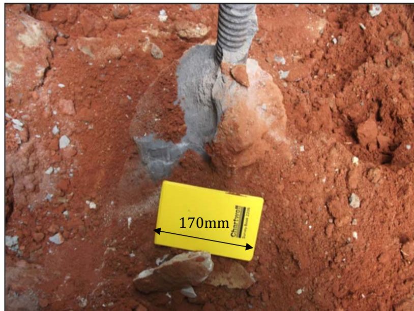
Figure 15. Exhumed top of constructed micropile.
