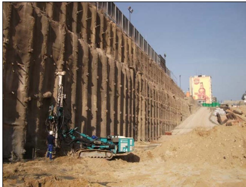
Figure 13. Pile Construction – South Wall.
