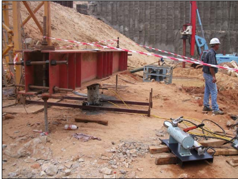
Figure 9. Pile Test Set Up.
