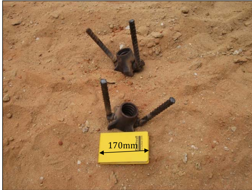
Figure 14. Typical Self drilled anchor heads for micropile construction.
