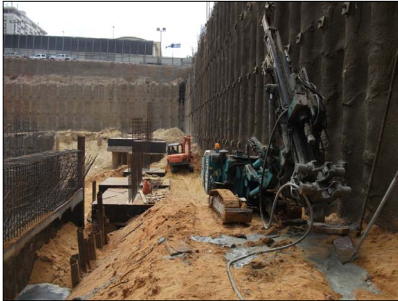
Figure 12. Pile Construction – North Wall.
