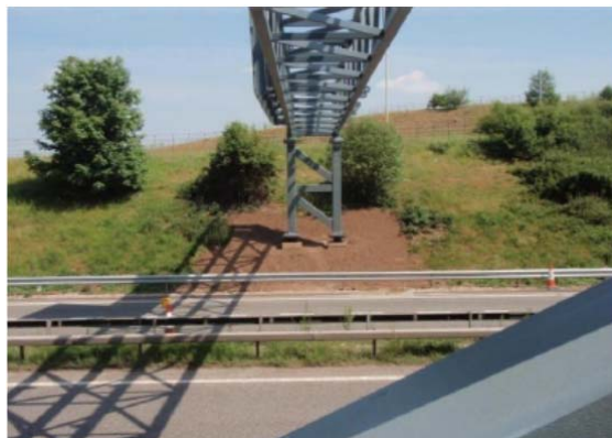
Figure 5. Highway Gantry, Motorway M4, UK founded with Micropiles
