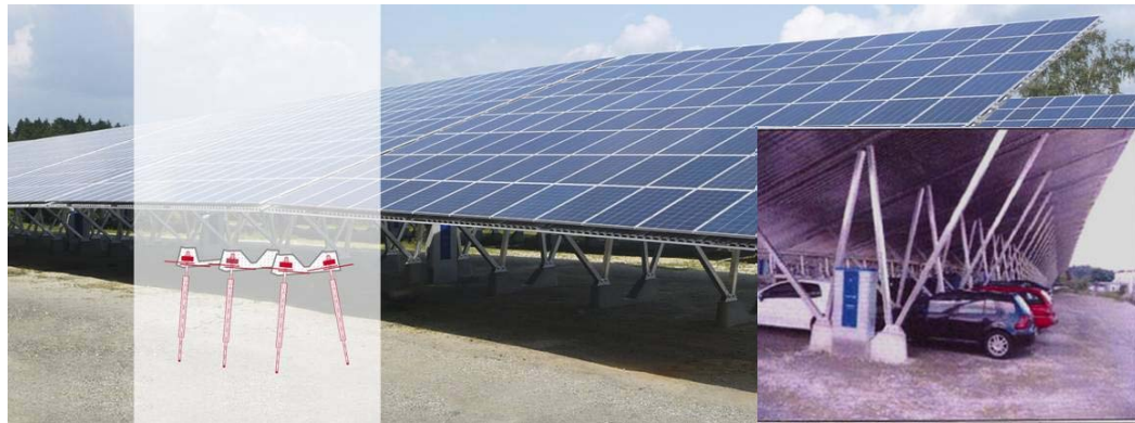
Figure 2. Solar Carport with deep foundation using drilled and pressure grouted TITAN 40/20 micropiles
