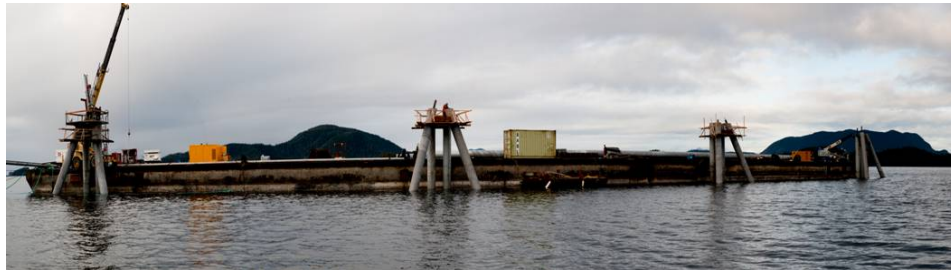
Figure 29. Jetty with Dolphins - reinforced with drilled TITAN 103/51 micropiles
