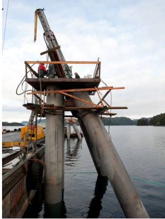
Figure 28. Dolphins from driven pipe piles – reinforced with drilled TITAN 103/51 micropiles
