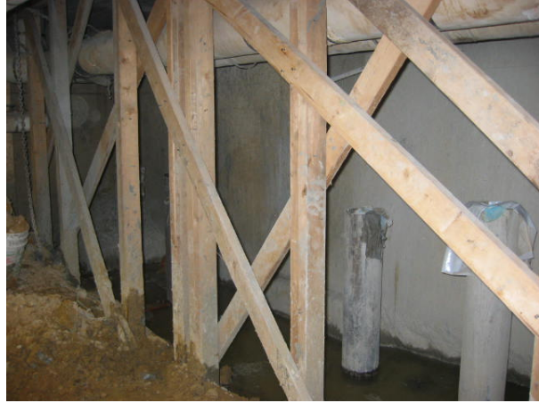
Figure 6. Core Holes through Floor Slab Figure 7. Shoring and Basement Micropiles
