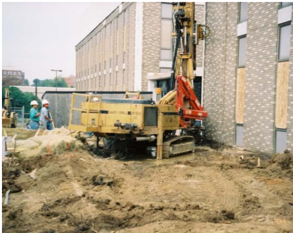
Figure 4. Perimeter Micropile Drilling
