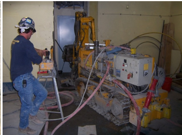
Figure 5. Interior Micropile Drilling
