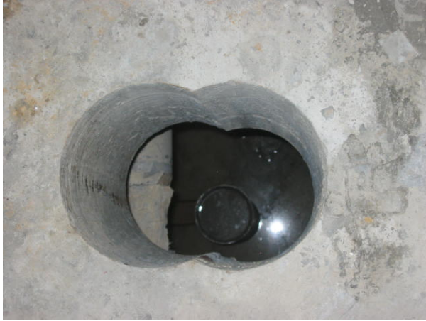
Figure 6. Core Holes through Floor Slab Figure 7. Shoring and Basement Micropiles
