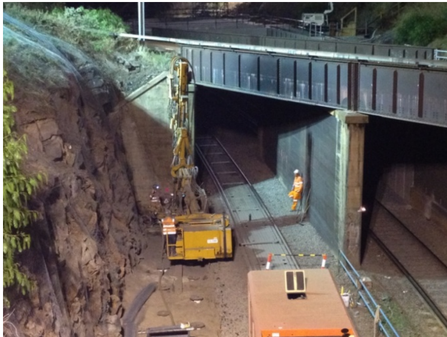
Figure 9: The Klemm predrilling the upper basalt
