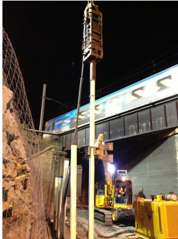
Figure 10: Piles were sequentially driven down until capacity was achieved.
