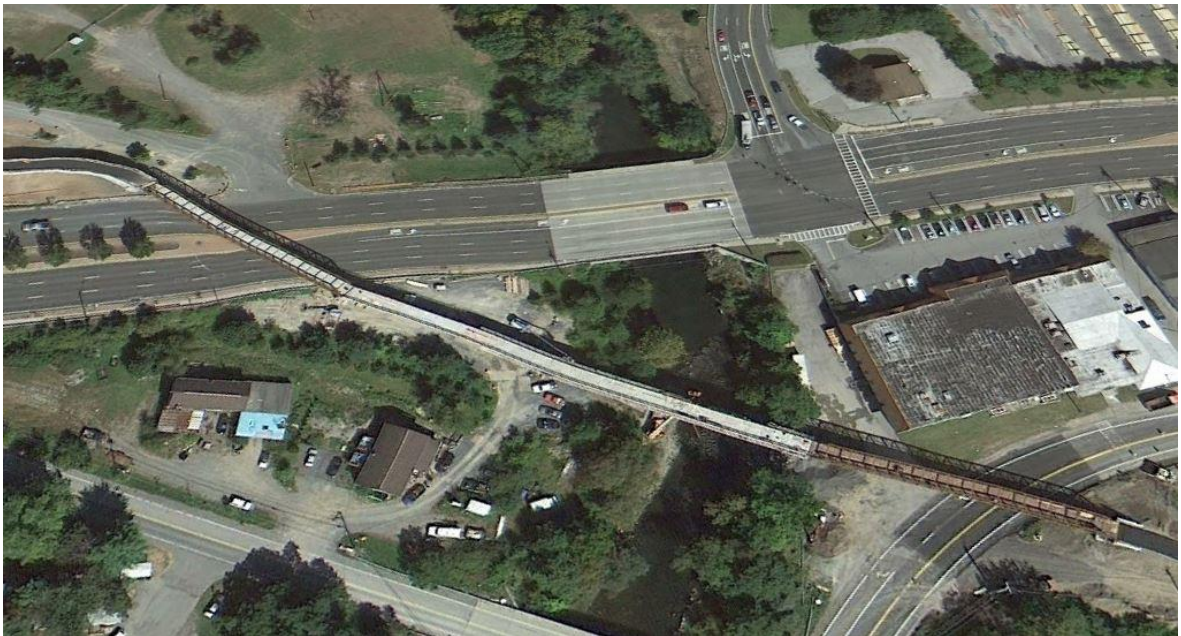
Figure 1. Aerial view of completed pedestrian bridges in Poughkeepsie, New York.
