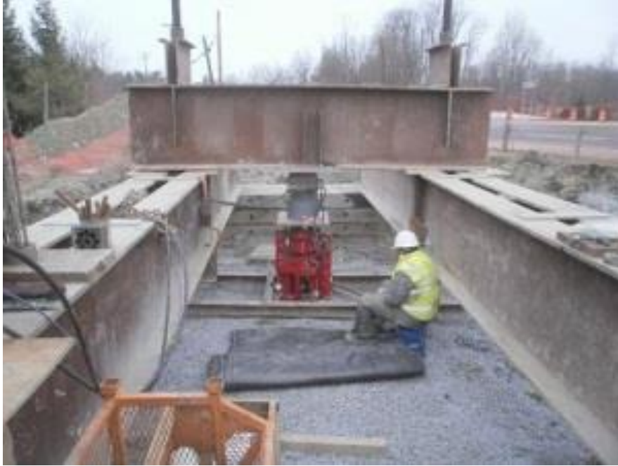
Figure 6. Picture of micropile load test setup
