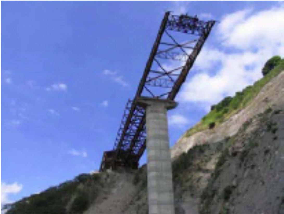
Figure 18. Launching girder.
