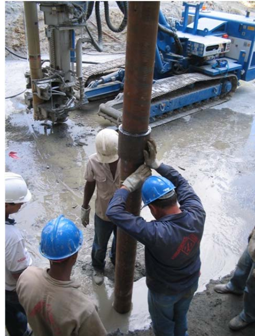
Figure 12. Installation of casing in grout-filled hole.
