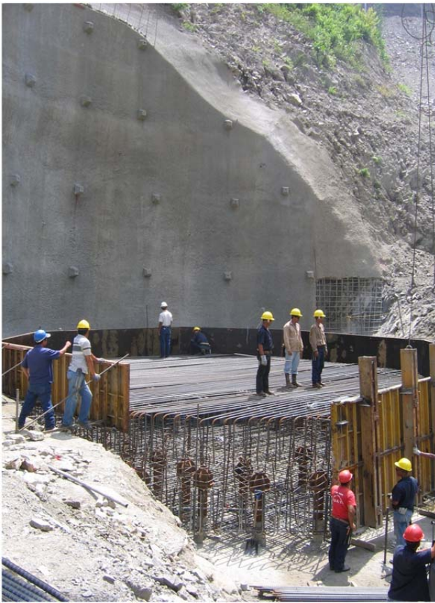
Figure 14. View of pile cap construction.
