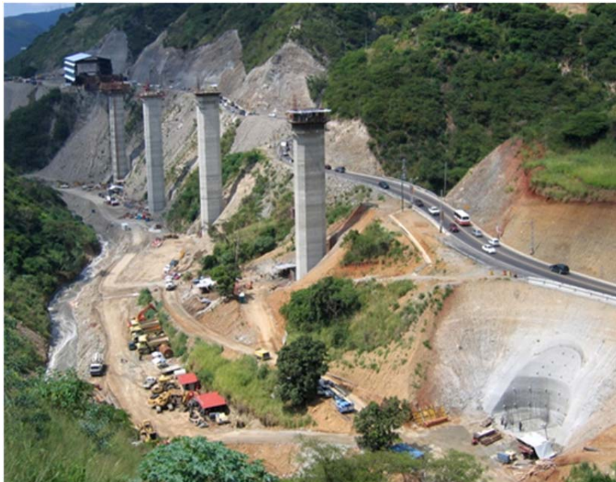
Figure 17. Simultaneous foundation, pilaster, and girder installation.
