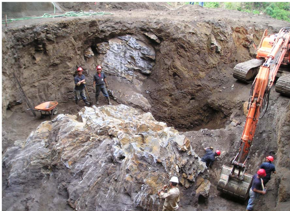
Figure 3. Ground conditions uncovered in an excavation for pilaster foundation.
