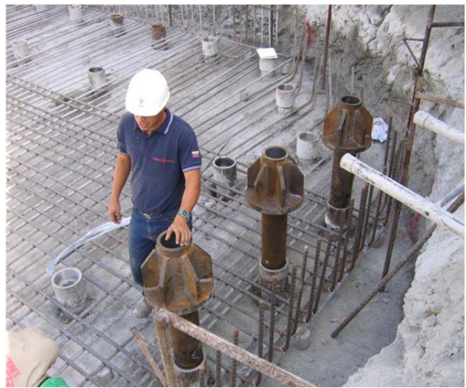
Figure 15. Connection of micropile-to-pile cap.
