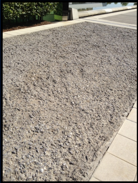
Concrete Road in Wroclaw
