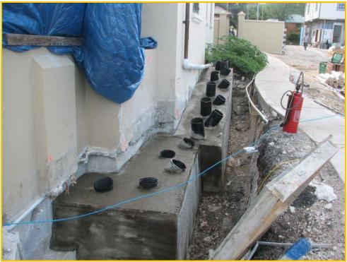
Figure 9: New Grade Beam around Foundation
