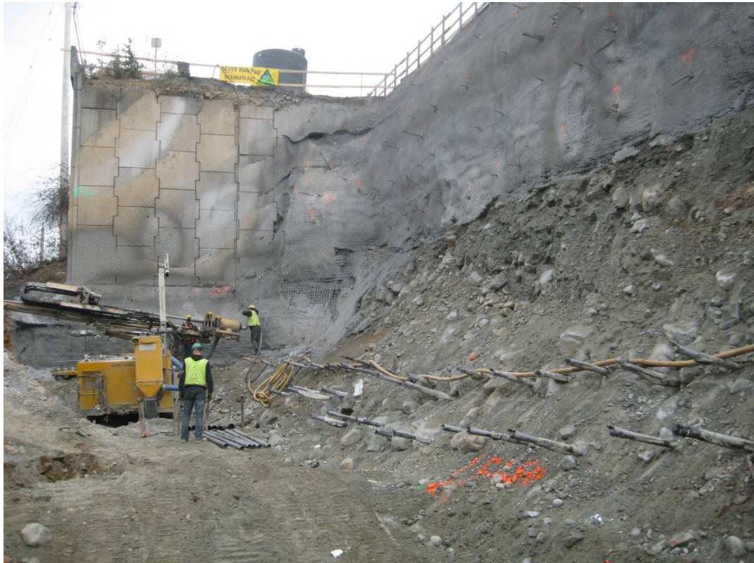
Figure 18. Installing the anchors to the footing of the new highway.
