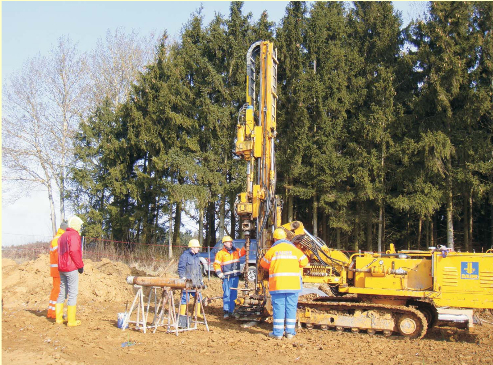
Drilling at the test site Mundlfing
