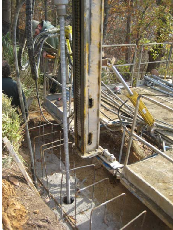
Figure 7. Installation of hollow core bar micropiles for tie beam.
