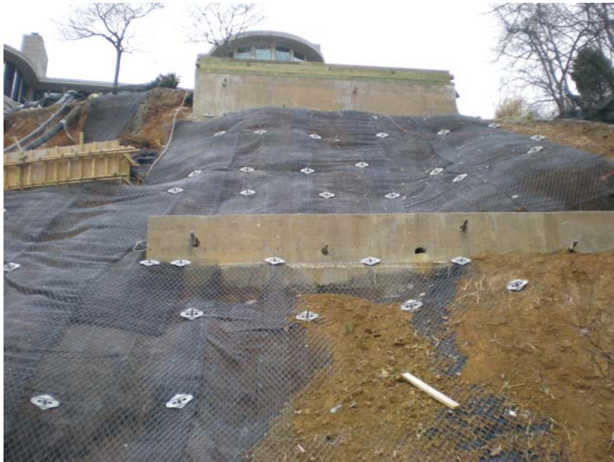
Figure 8. Completed tie beams on the northern end of the slope.
