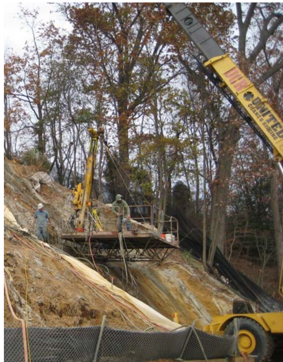
Figure 6. Crane-suspended mast for micropile installation
