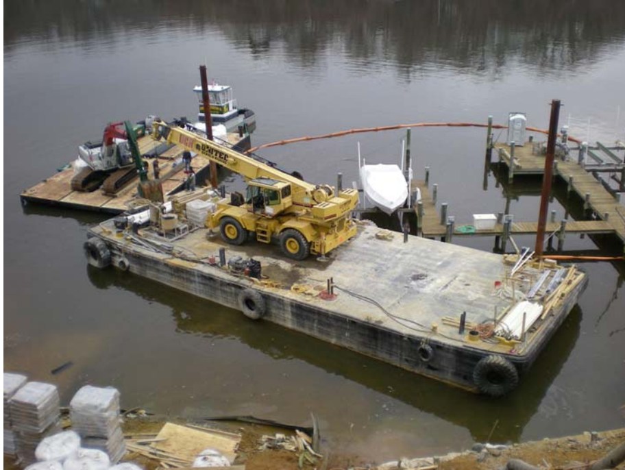
Figure 5. Barge arriving on site with crane and supplies.
