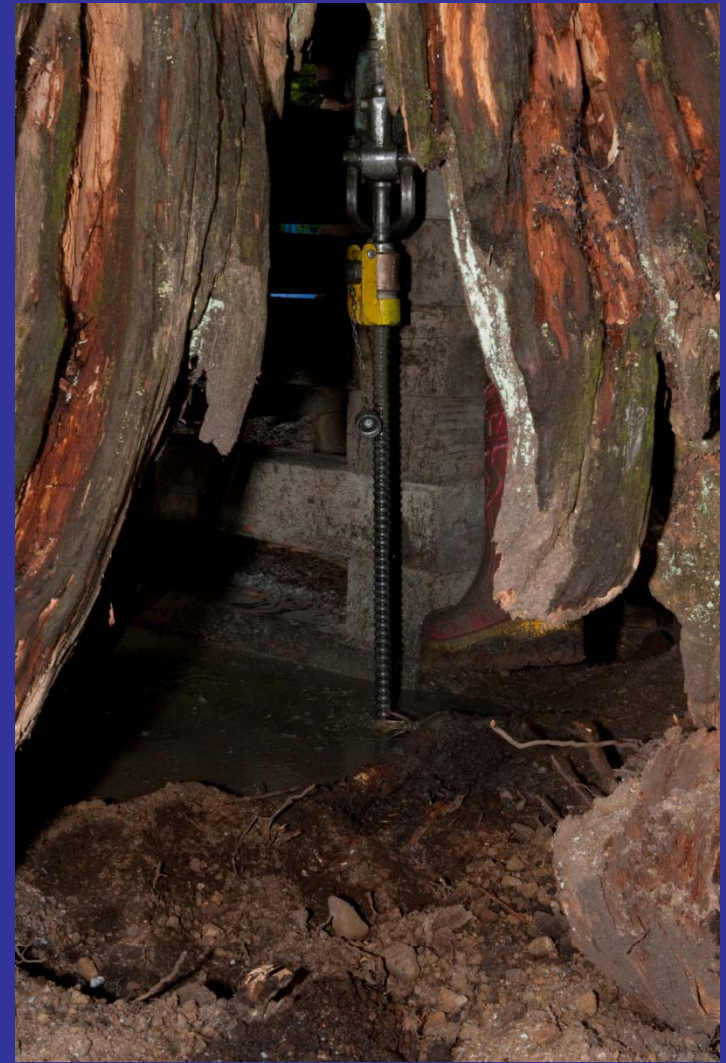
IBO (Injection Boring) Titan Micro Piles (Root Piles) installed with a hand held Drill inside the hollow tree
