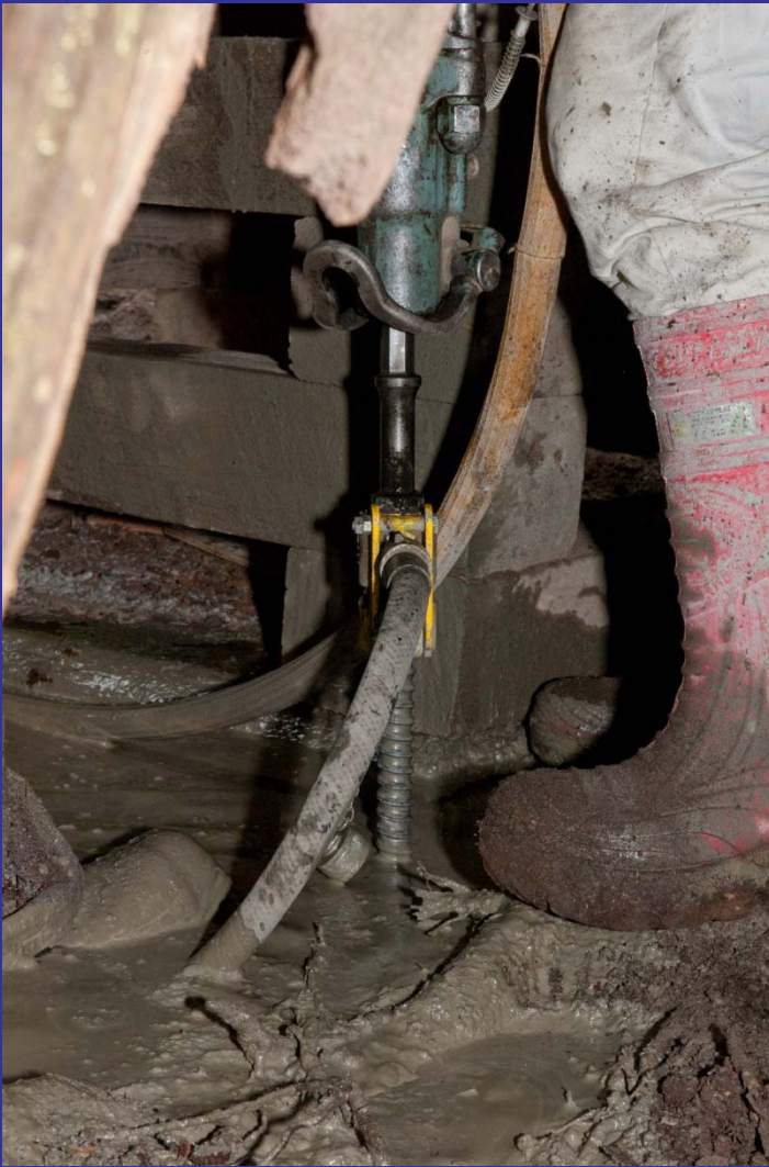
IBO (Injection Boring) Titan Micro Piles (Root Piles) installed with a hand held Drill inside the hollow tree
