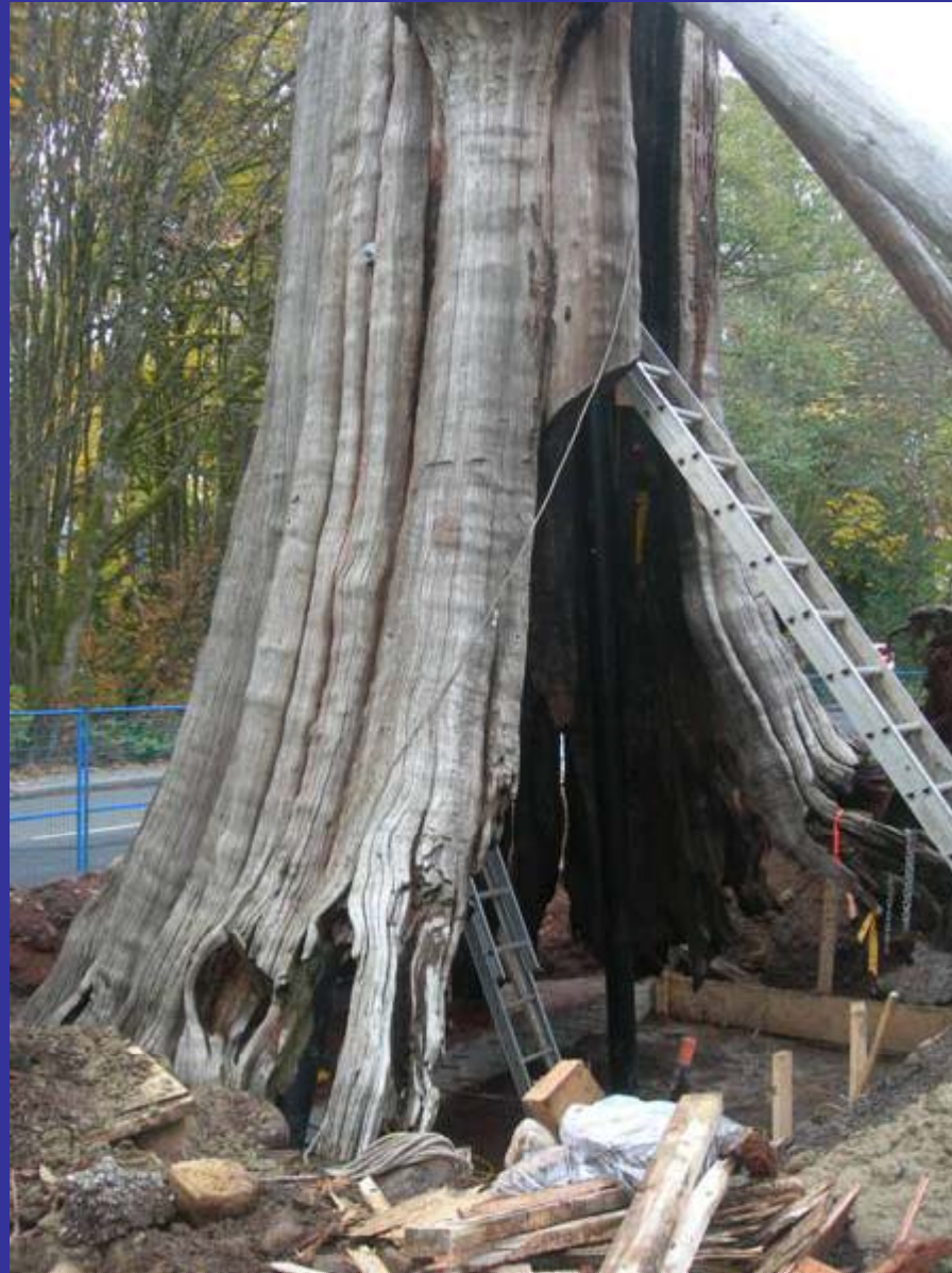
Before placing Pile Cap Concrete
