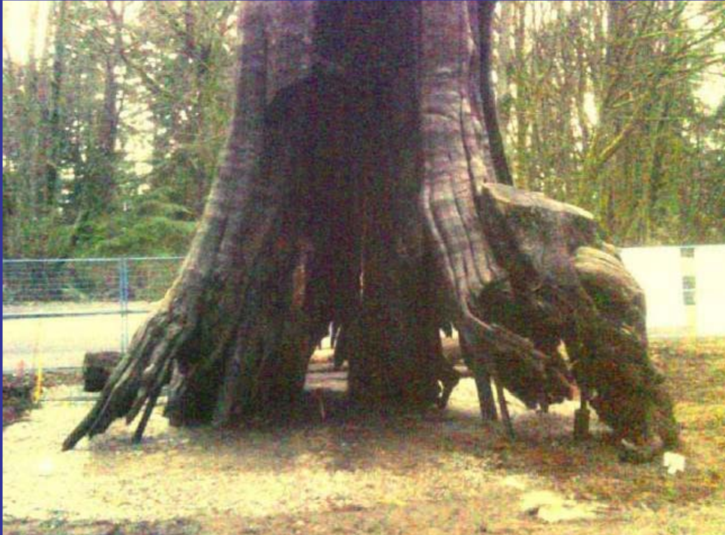
The tree now connected to the Root Piles before the landscaping
