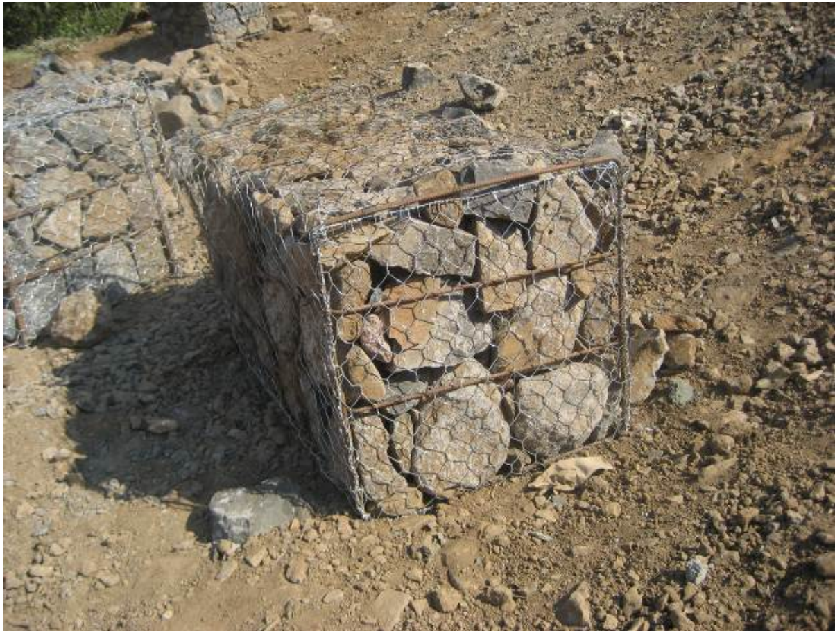
11 stone filled gabions
