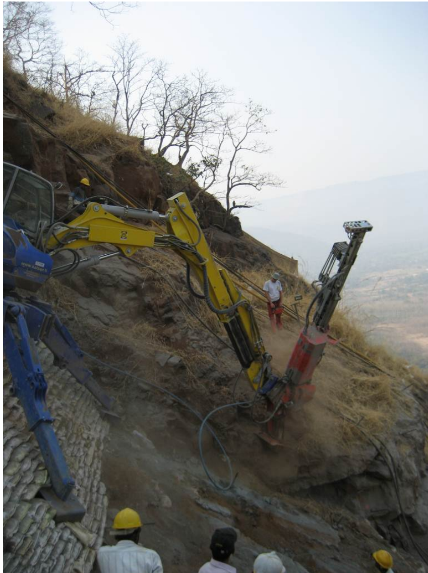
12 drilling from walking dragline slope 2
