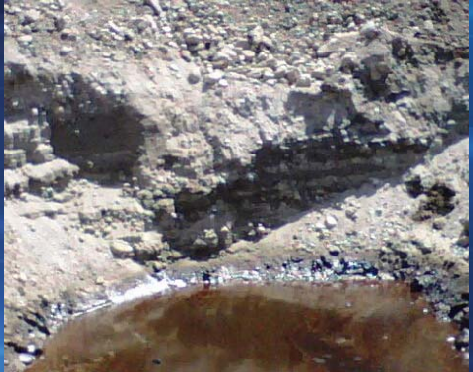
5 m Excavation in Dredged Fills
