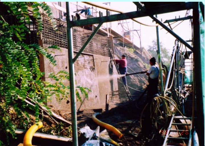
Spraying of wall
