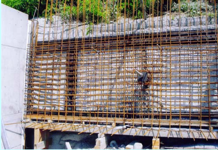
Installation of reinforcement and anchor heads
