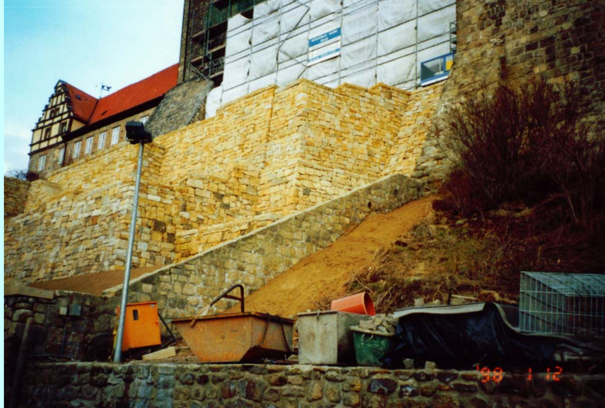
Front view of completed fully faced wall section
