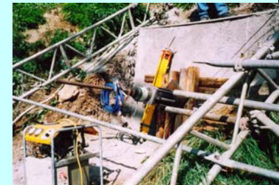
Static load tests
