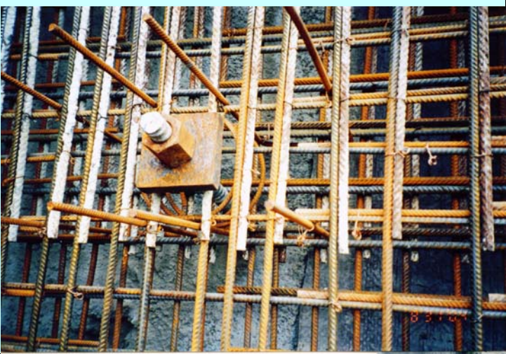
Anchor head detail
