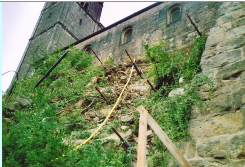
Anchor in the slope
