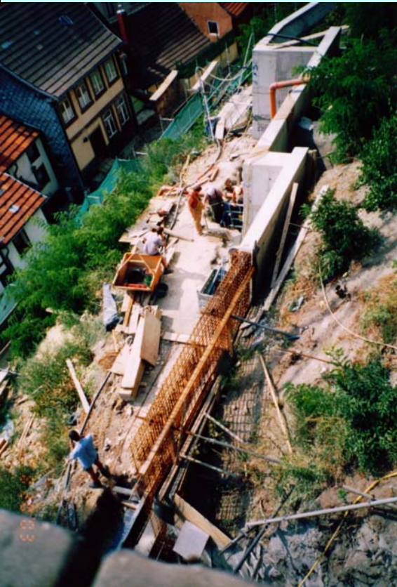
Wall sections from above
