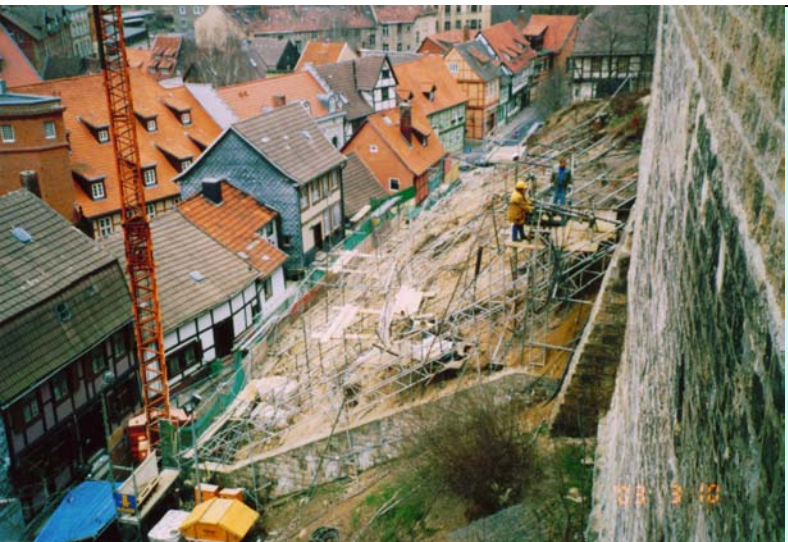
Installation of anchors from a light scaffolding platform
