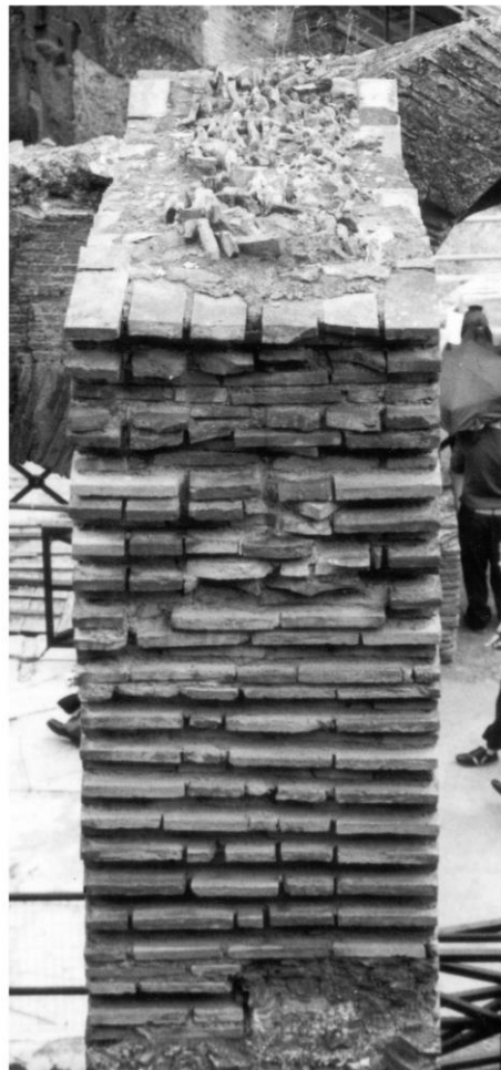
Figure 1. Rubble In-fill Wall. Colosseum. Rome.
