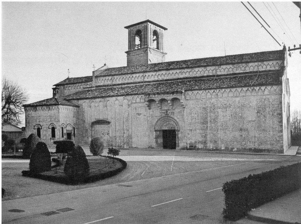
Figure 19. Spilimbergo Cathedral. Retrofitted Structure 2 .
