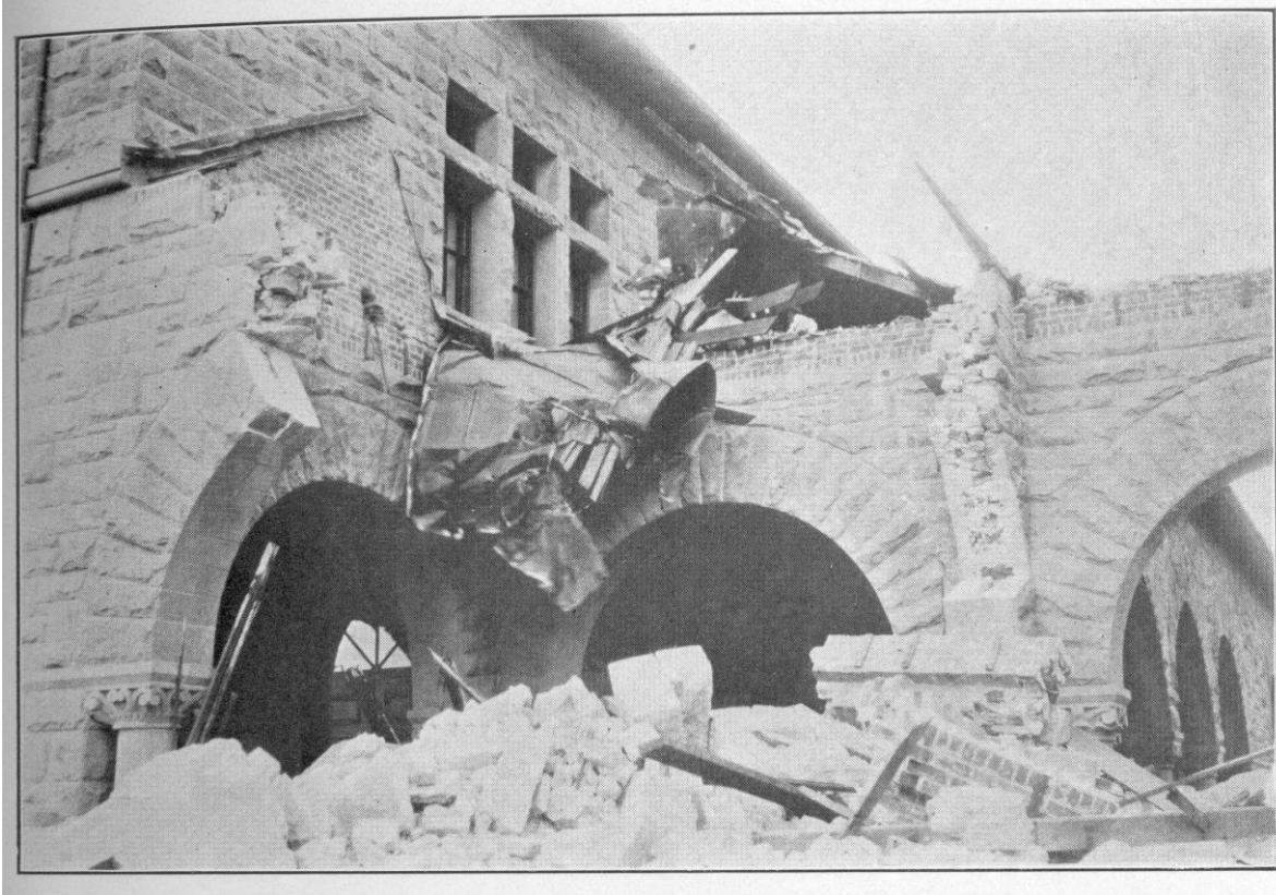
Figure 2. Stanford University. 1906 Earthquake Damage to URS Arch 2 .
