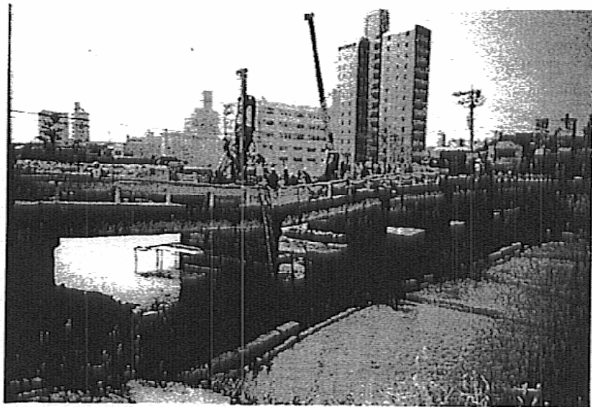
Photo-3 The Construction Situation
