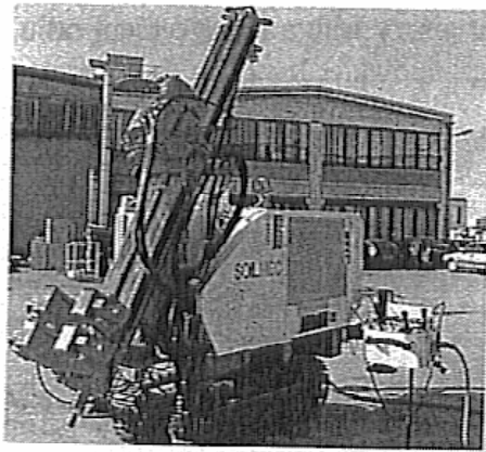
Photo. 4 Drilling machine (SM103)
