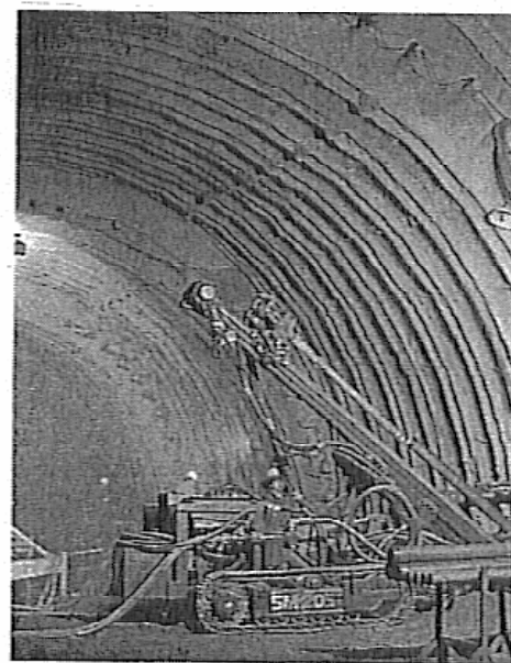
Photo.1 Micropiling operation
